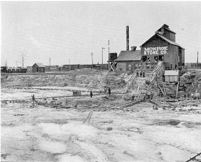
Plate IV. Monroe Stone Company, crusher and west wall of quarry.
