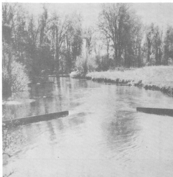
Figure 62. Jetties deflect eroding currents and arrest the decay of stream banks.
