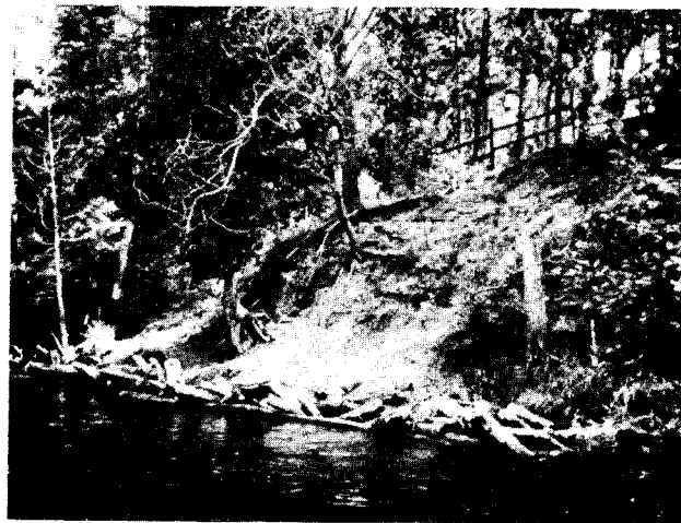
Figure 68. Rip rap of logs and stumps protects the base of a high sandy bank at this campsite on the Au Sable below Grayling. Upper slope is eroding because some campers still climb up and down banks to enter and leave the river.
