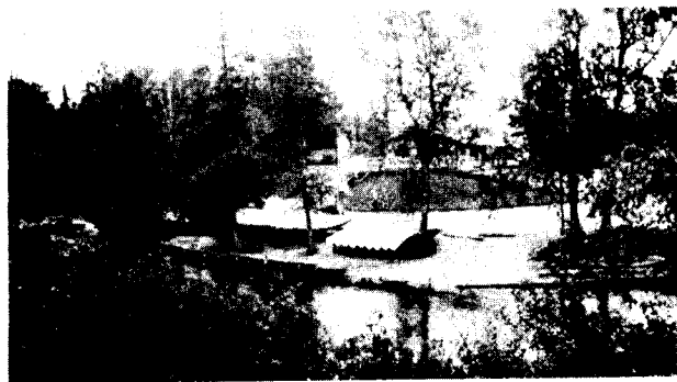
Canoe Livery landing on Manistee River. Bank is protected by wood sheet piling for boat dockage.
