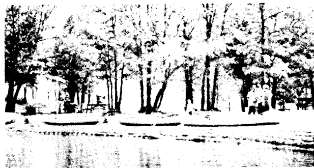
Canoe landing in Au Sable River at Canoe Camp protected by concrete ramp. However, most canoes land upstream from ramp on unprotected bank.
