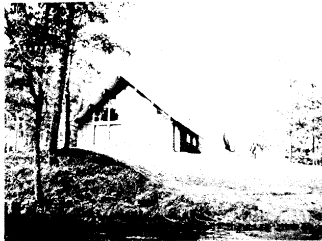
Grading the lot at this cabin allows silt and sand to wash into the river.
