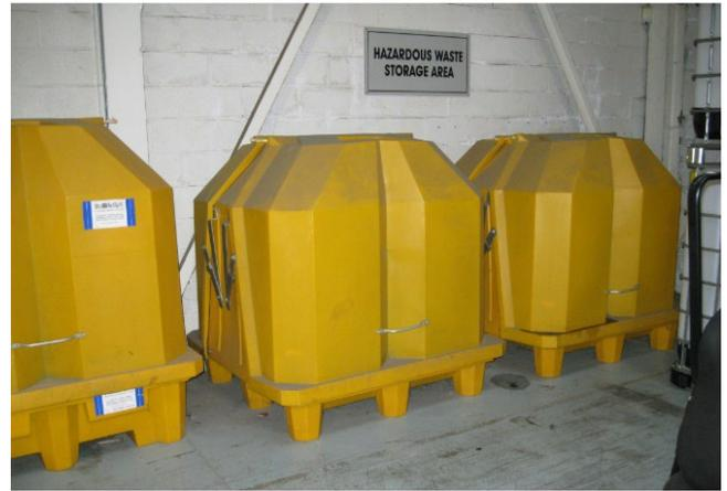
Four drum lockable secondary containment cabinets with squirt control
