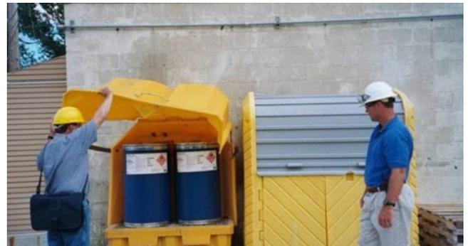
Two drum lockable secondary containment cabinets with squirt control
