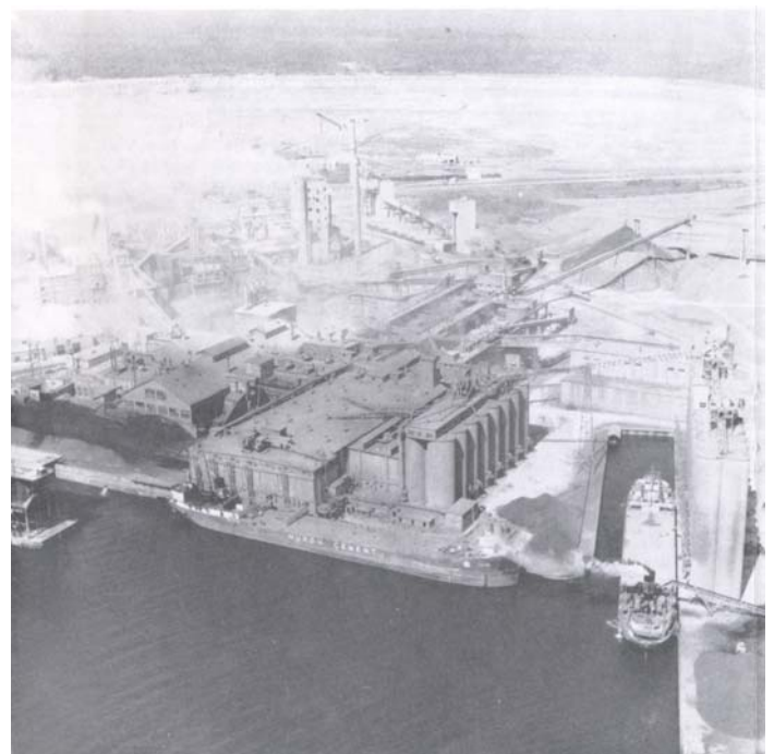
Photo 3. Huron Portland Cement Company, subsidiary of National Gypsum Co., Alpena, Michigan. Aerial view looking west.
