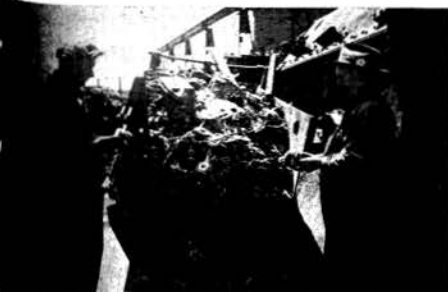
Fred Faller and Richard Bree, separating leached motor parts for ship bottom paint.
