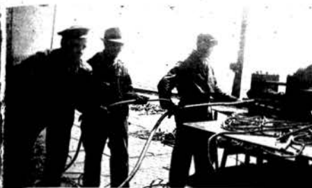
Carl A. Delro, Edmund Emond and Leo Jolly, stripping insulation from armored navy cable.
