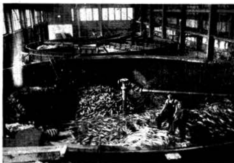
Ray Dussault and Frank Brula, loading secondary copper into tank for leaching at Tamarack Reclamation. Subdivided tank for treating lots separately, shown in background.
