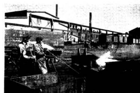
Roy Matson and James Zubiena, burning insulation and grease from motor parts.
