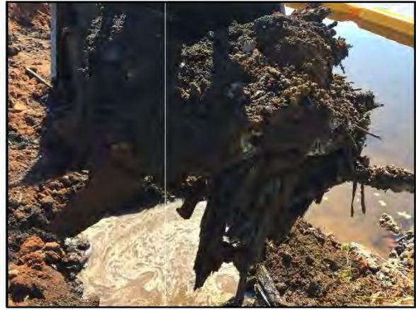
Photo 8: View of white sludge material mixed with sediment, excavated from shoreline as part of Container #10. Photo taken July 11, 2017.
