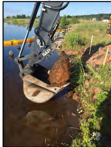
Photo 10: View of partial drum and hardened contents removed from shoreline during excavation. Photo taken on July 11, 2017.
