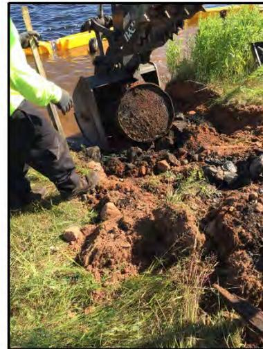
Photo 4: View of submerged Container #1 (DM-04) being removed from shoreline during excavation. Photo taken July 10, 2017.
