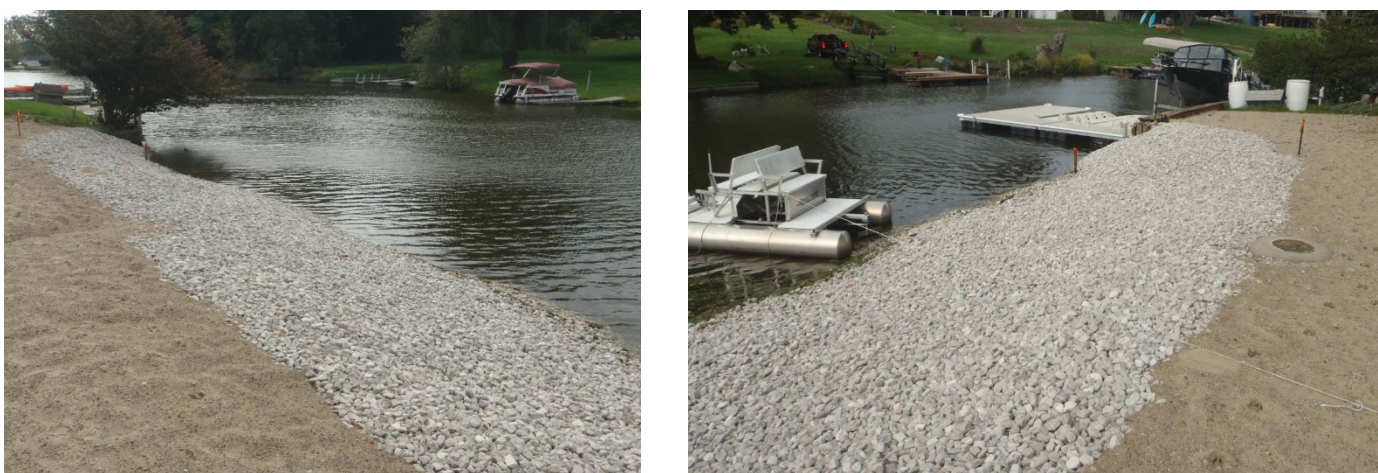
Figure 6. Fenner's Ditch facing west, October 2018 site evaluation.
