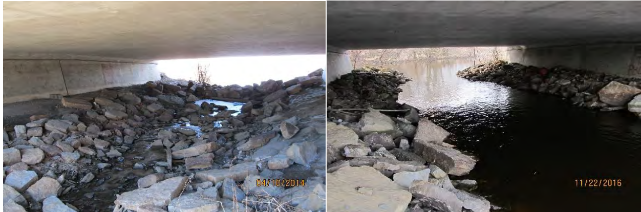
Channel under Ogden Street, before and after removal of excess riprap and debris (C. Bougie, WDNR).
