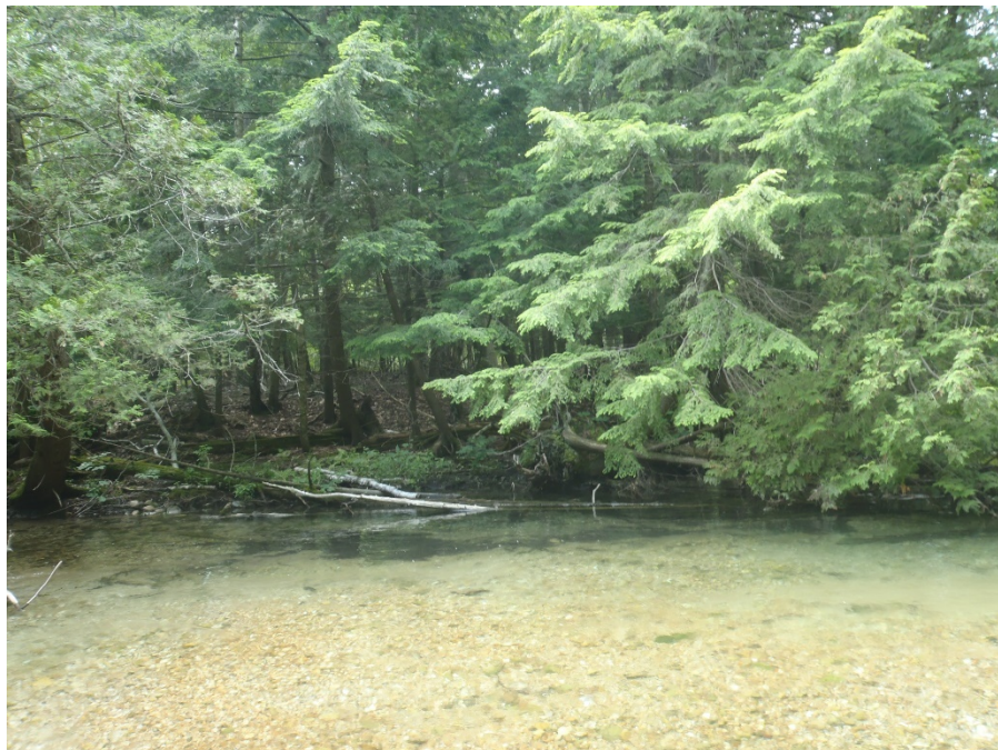
Figure 26. Sand deposition and widening pool upstream of County Road 675, caused by water not flowing properly through the culvert. Crystal River, Leelanau County, Michigan, July 2018.
