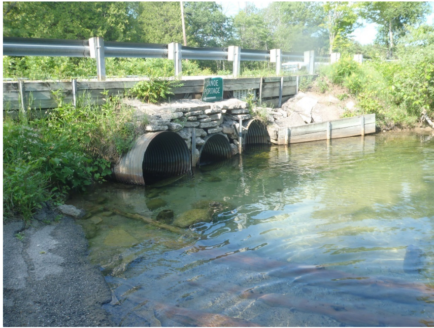
Figure 25. Road Crossing at County Road 675, Crystal River, Leelanau County, Michigan, July 2018.
