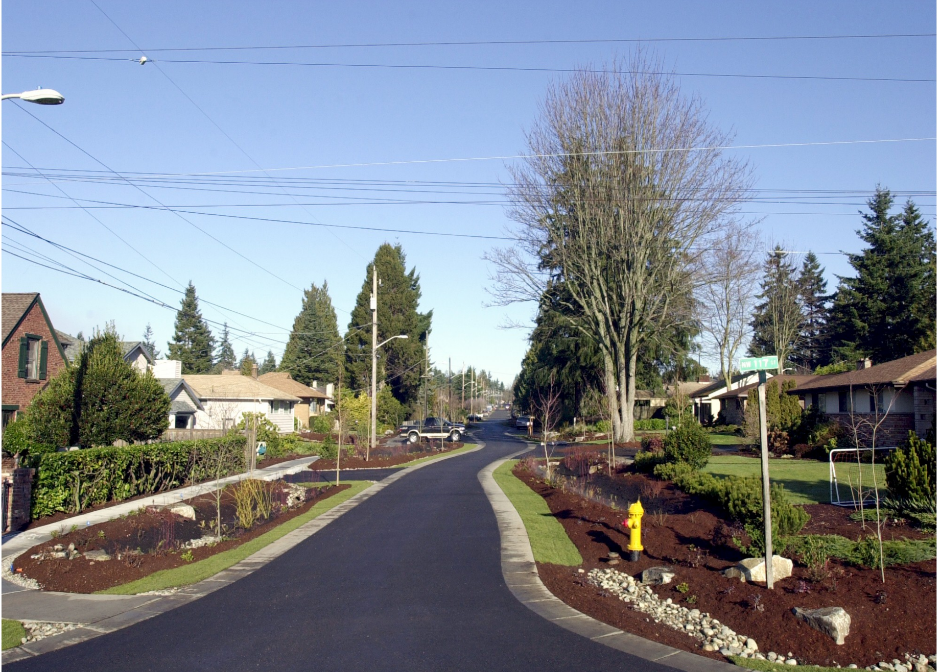
After Completion - January 2001
