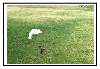
Garfield Street Before: The septic tank on this site was structurally compromised and the drain field was saturated. This caused both surface discharge and groundwater discharge of untreated sewage into the nearby creek.
