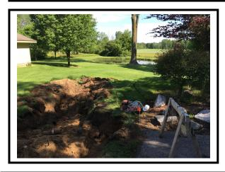
Warner Street Before: The drain field on this site was in failing condition. It was not properly treating effluent, causing untreated waste water to drain into the nearby creek.
