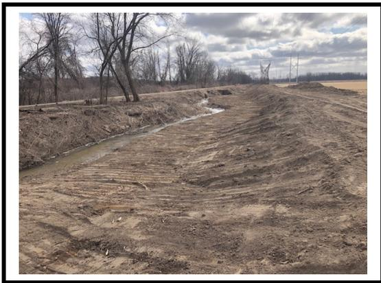
**Project area 5: Two stage ditches were installed to address streambank erosion, falling trees, etc.**
