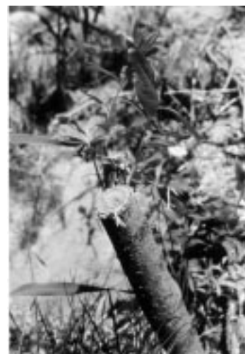
Picture 3, left, shows a fascine, brush layering and live stakes. Picture 4, below, shows new growth from a live stake. Source: Whetstone Creek Nonpoint Source Watershed Project.
