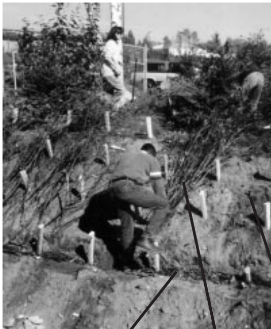
Picture 3, left, shows a fascine, brush layering and live stakes. Picture 4, below, shows new growth from a live stake. Source: Whetstone Creek Nonpoint Source Watershed Project.
