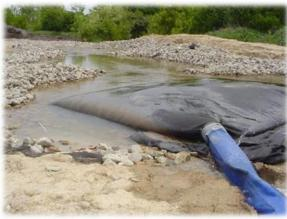
For very small sized sediment particles, such as fine silts and clay, polyacrylamides (PAMs) must be used in conjunction with other sedimentation controls such as filter berms, filter bags, sedimentation basins, geotubes, and geojute. PAMs bind with the sediment particles forming a flock that settles out of the water column.
