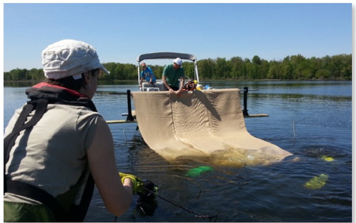
Divers deploying a natural fiber benthic barrier.
