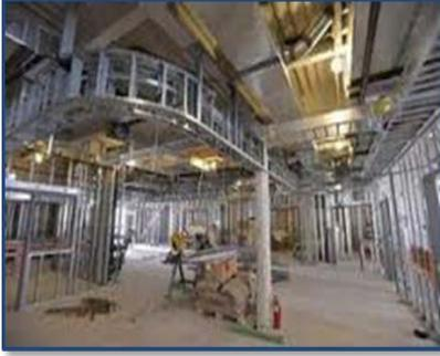
While conducting a project inspection, fire marshal inspectors survey and inspect for proper installation and maintenance of fire protection features, such as fire alarm and detection systems, fire suppression systems, fire separation and fire barriers/compartments, means of egress, interior finish and emergency power.
