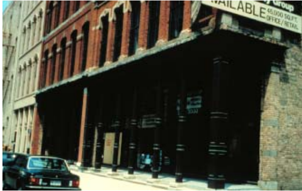
Cast-iron columns providing structural support for exterior wall
