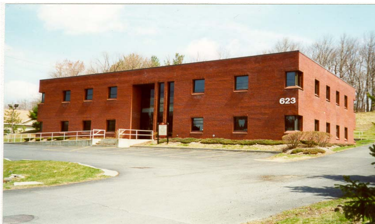
Protected steel frame structure
