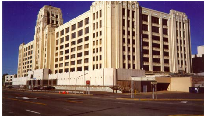
Concrete framed structure
