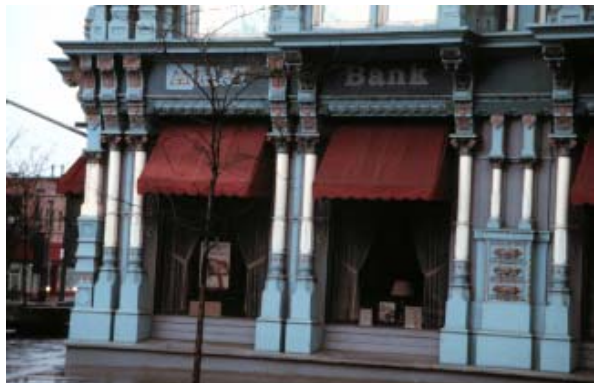
Cast-iron building front providing structural support to exterior wall of building
