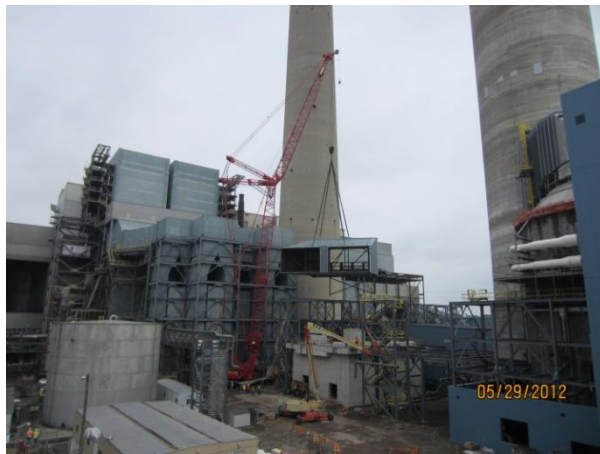
Implementation of Critical Lift Plan
