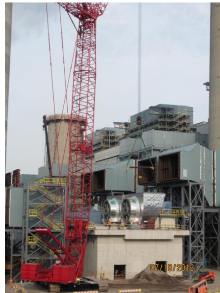
Proper Rigging Techniques
