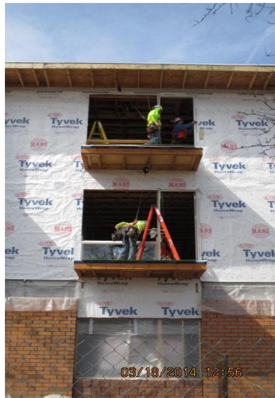
Carpenter's tied-off while installing balcony windows & doors
