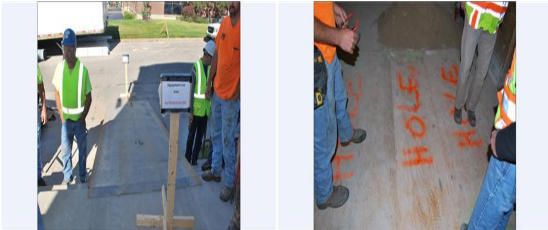
Pictures: Ramp signs and secured hole covers throughout the site
