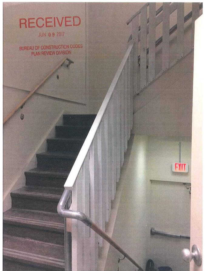
Guard and Handrail Modified Center Stair
