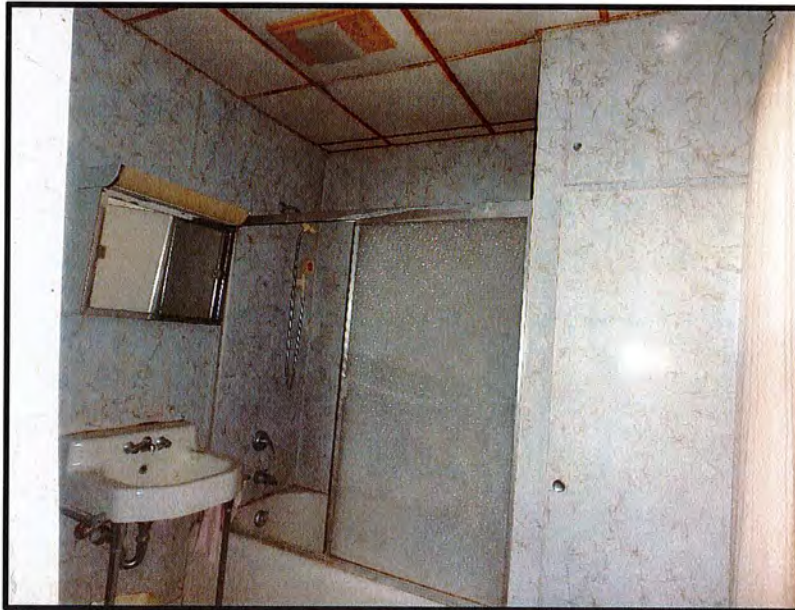
INTERIOR VIEW OF BATHROOM (FS-10)
