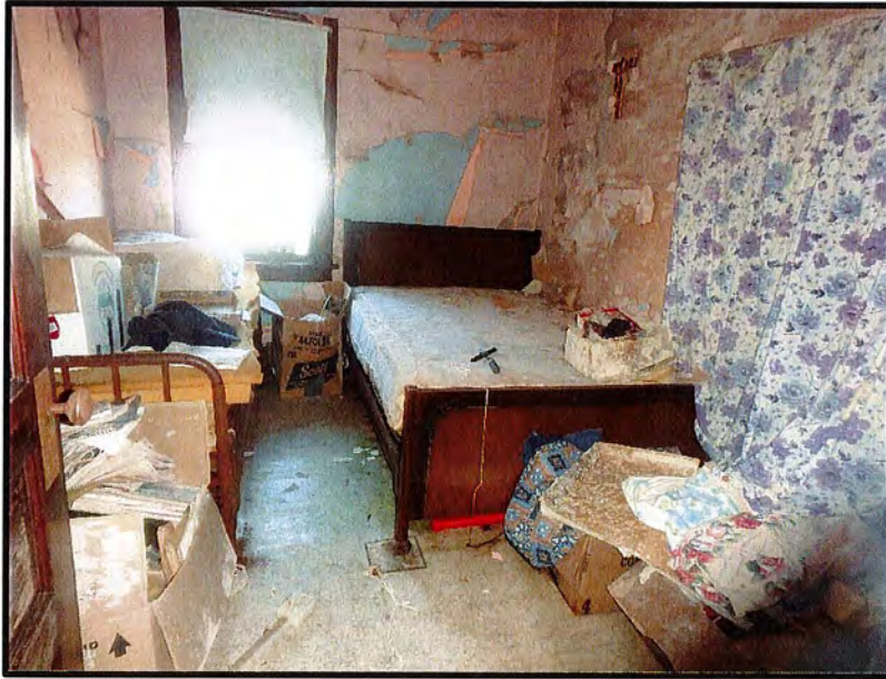
INTERIOR VIEW OF BEDROOM #1 (FS-3)
