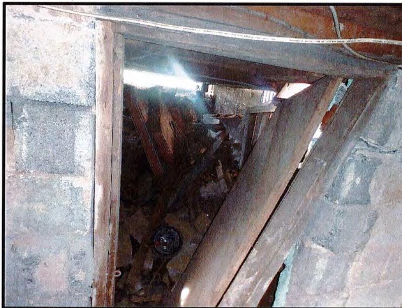
EXTERIOR VIEW OF BASEMENT (FS-10)
