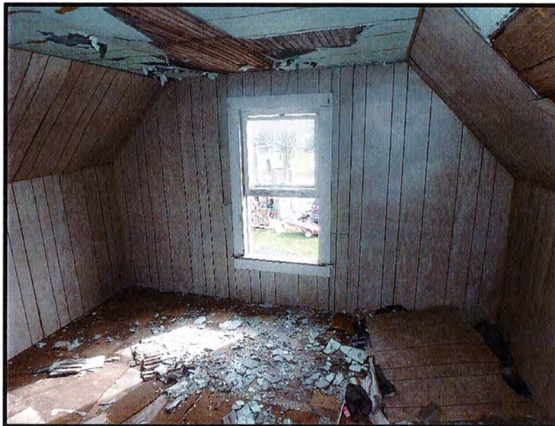
INTERIOR VIEW OF 2 nd FLOOR (FS-8)
