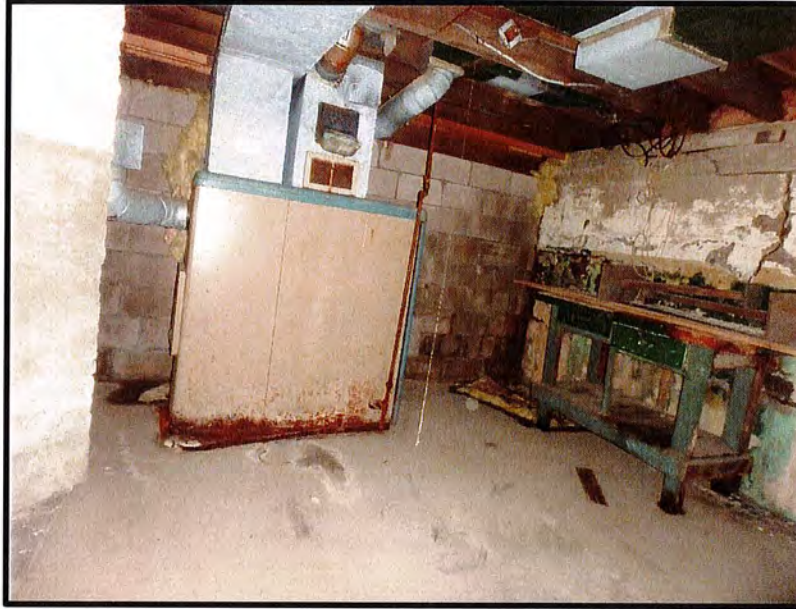
INTERIOR VIEW OF BASEMENT (FS-7)
