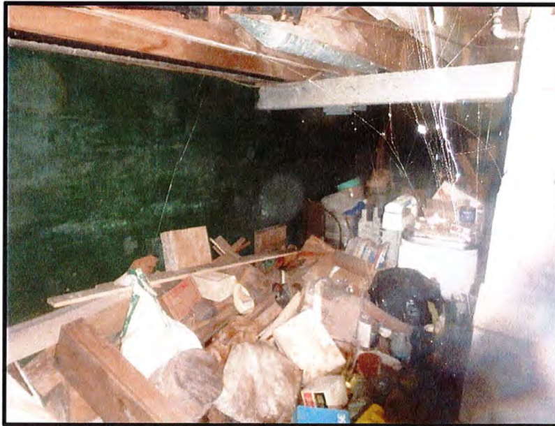
INTERIOR VIEW OF BASEMENT (FS-9)
