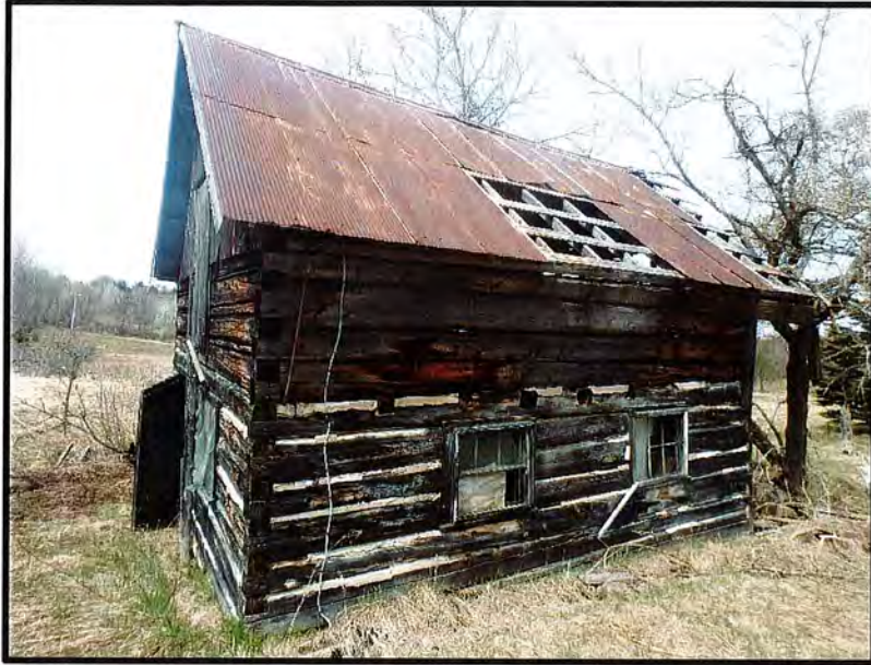
EXTERIOR VIEW OF BARN (FS-17)
