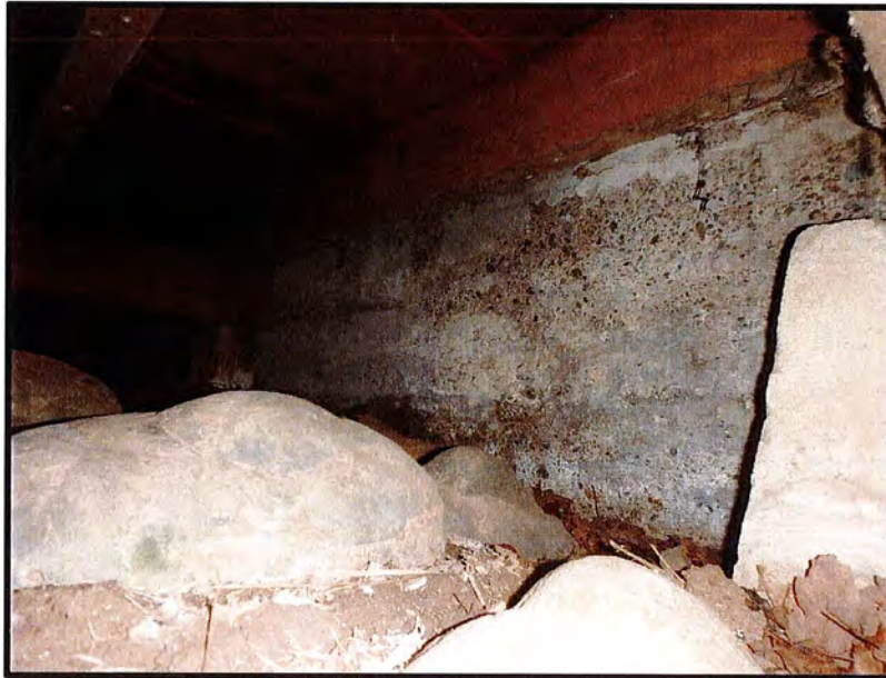
INTERIOR VIEW OF CRAWLSPACE (FS-12)
