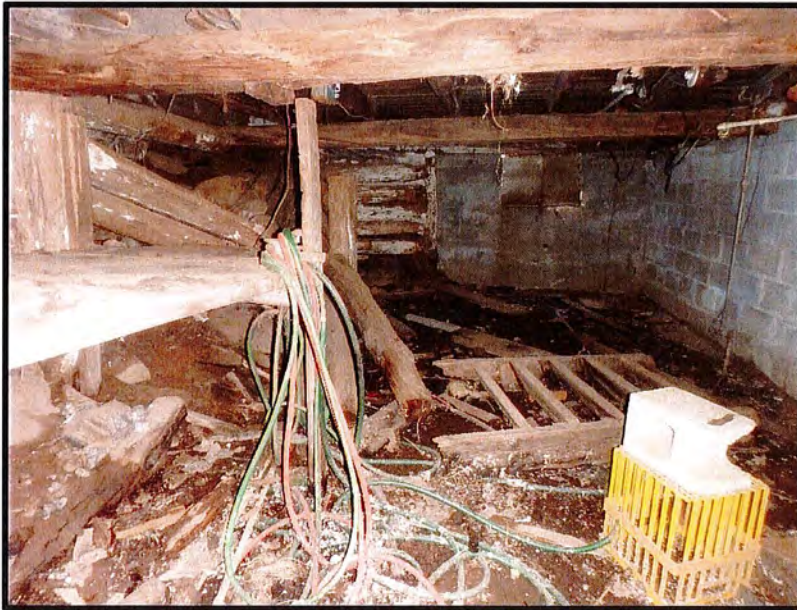
INTERIOR VIEW OF BASEMENT (FS-13)
