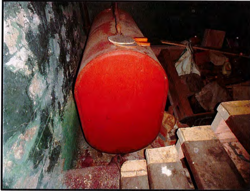
INTERIOR VIEW OF BASEMENT (FS-9) SHOWING OIL TANK
