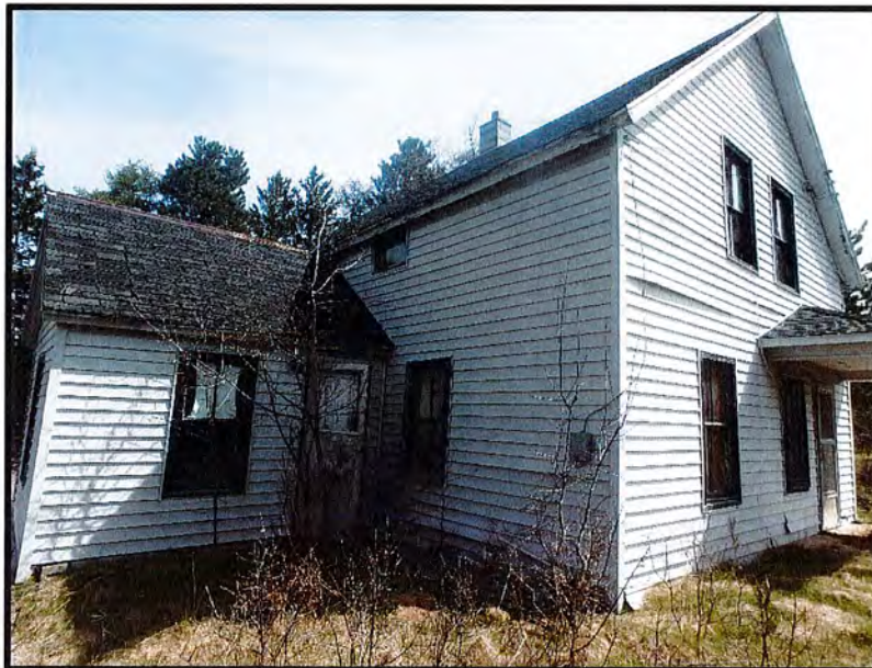
EXTERIOR VIEW OF HOUSE FACING NORTHEAST
