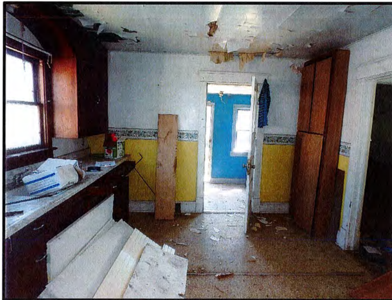
EXTERIOR VIEW OF KITCHEN (FS-2)
