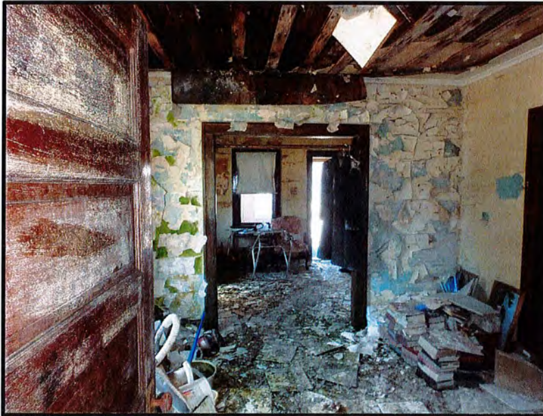
INTERIOR VIEW OF DINING ROOM (FS-4)
