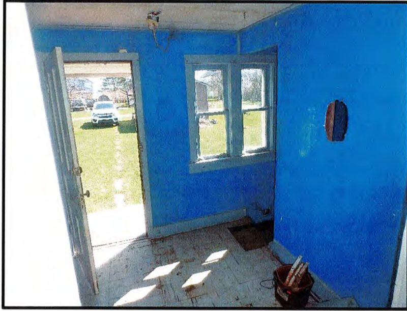
INTERIOR VIEW OF UTILITY ROOM (FS-5)
