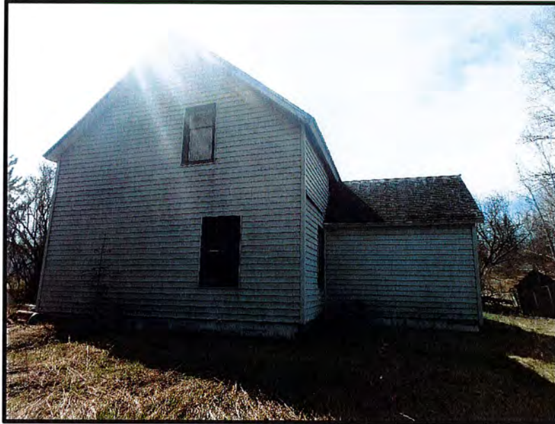
EXTERIOR VIEW OF HOUSE FACING SOUTH
