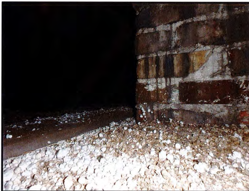
INTERIOR VIEW OF ATTIC SHOWING VERMICULITE AND PERLITE INSULATION (FS-9)
