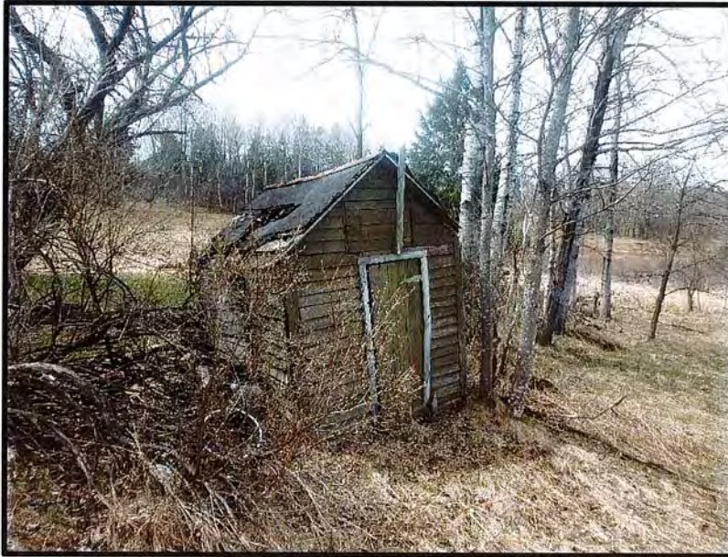
EXTERIOR VIEW OF OUTHOUSE (FS-16)
