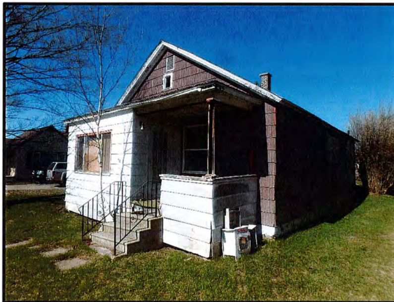
EXTERIOR VIEW OF HOUSE FACING SOUTHEAST
