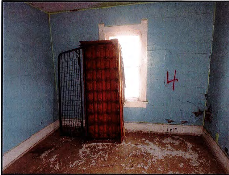
INTERIOR VIEW OF BEDROOM (FS-4)
