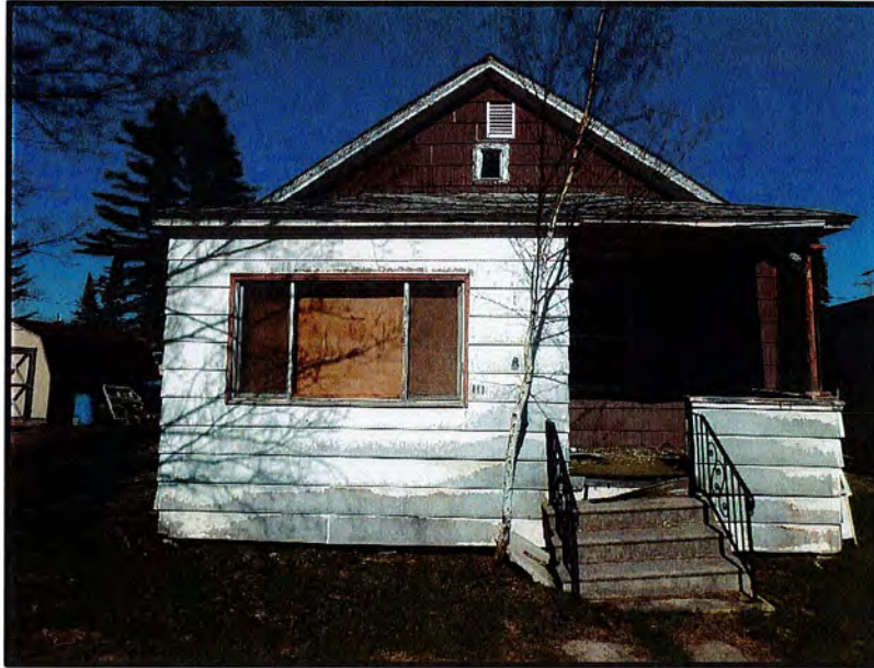
EXTERIOR VIEW OF HOUSE FACING SOUTH
