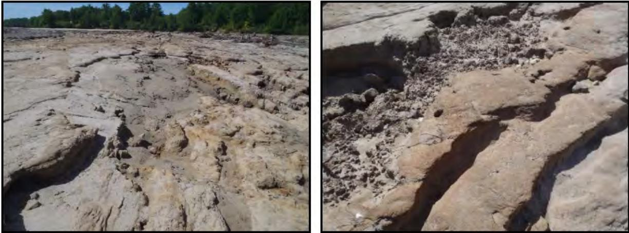
Figure 4 Reservoir bed scouring.
