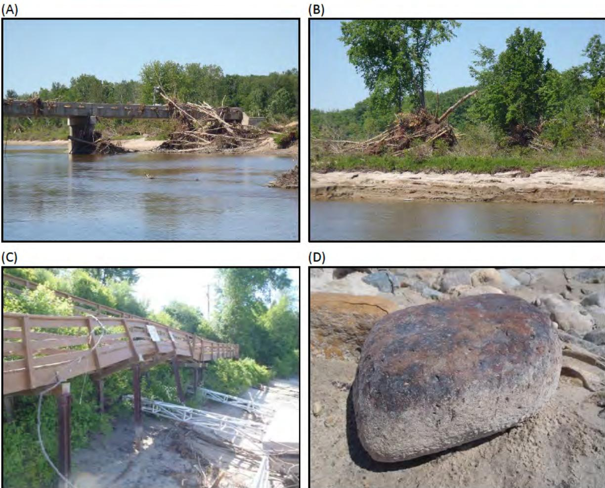
Figure 5 Indicators of reservoir bed scour. (A) and (B) flood debris above the regular reservoir water level. (C) Damage to infrastructure, above the regular reservoir water level. (D) Dark iron or manganese sulfide coating on the upper side of a large rock, indicating the rock was flipped over by hydraulic conditions during the reservoir drawdown.
