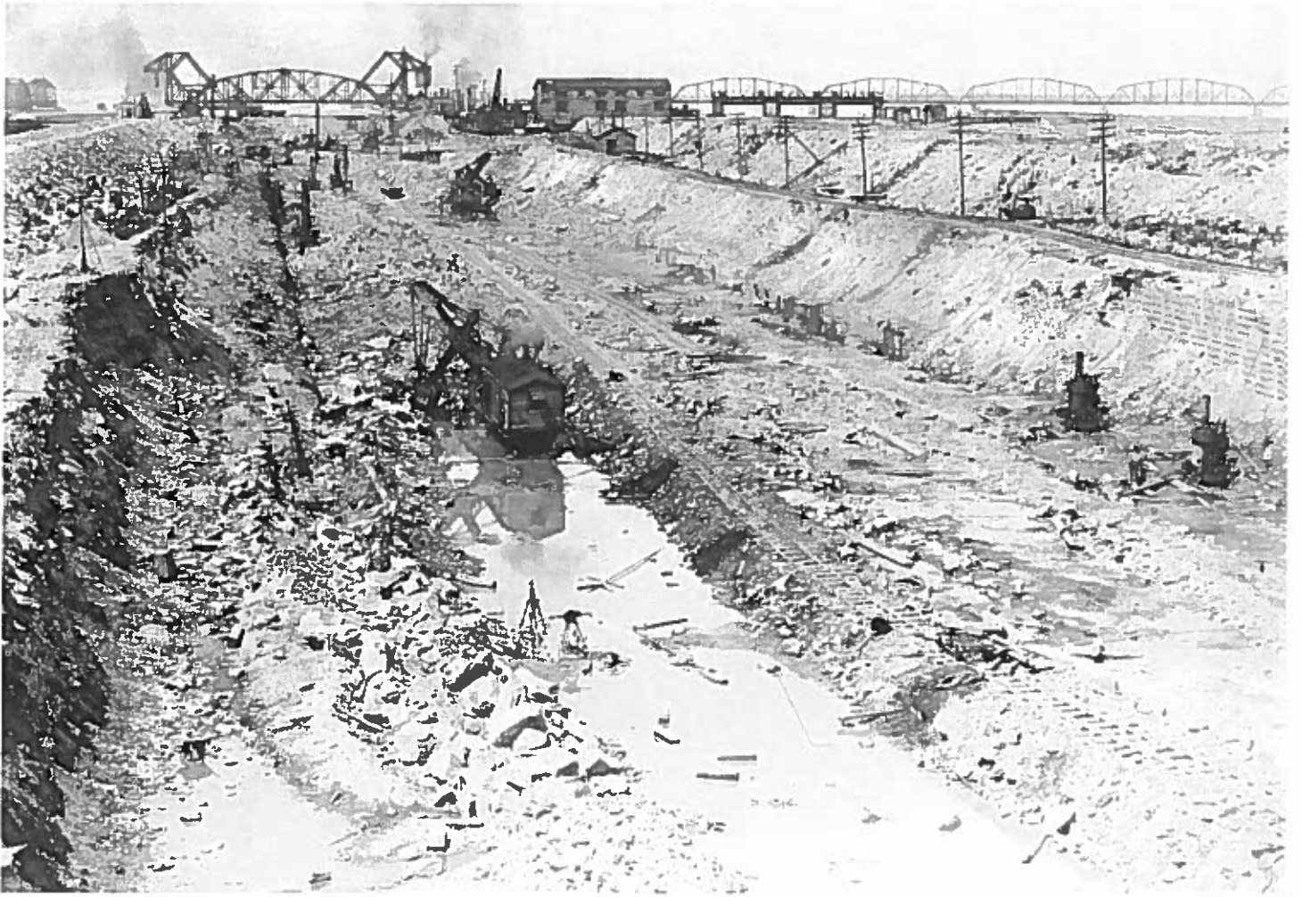
Excavation of the Davis Lock, early 1900's.
