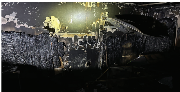
Image of wall where electrical fire is believed to have started
