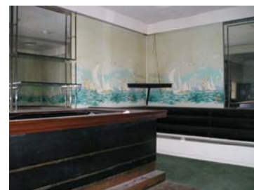
Picture right shows a bar which is in fair condition.
