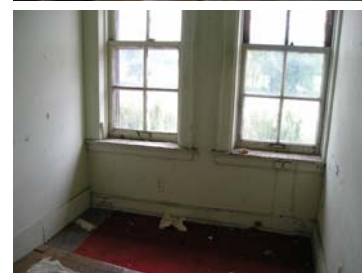
Picture left shows the River room extension which has been recently refurbished. The acoustic ceiling tiles, walls and carpeting are in fair condition. Picture shows a window with wooden window frames in poor condition.
