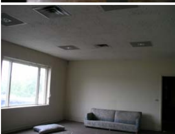
Picture left shows the River room extension which has been recently refurbished. The acoustic ceiling tiles, walls and carpeting are in fair condition. Picture shows a window with wooden window frames in poor condition.
