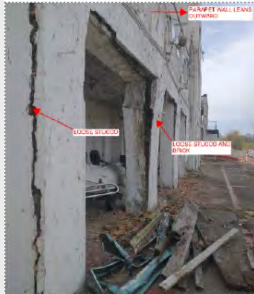
Photo No. 13 – North terrace, east end, exterior wall
