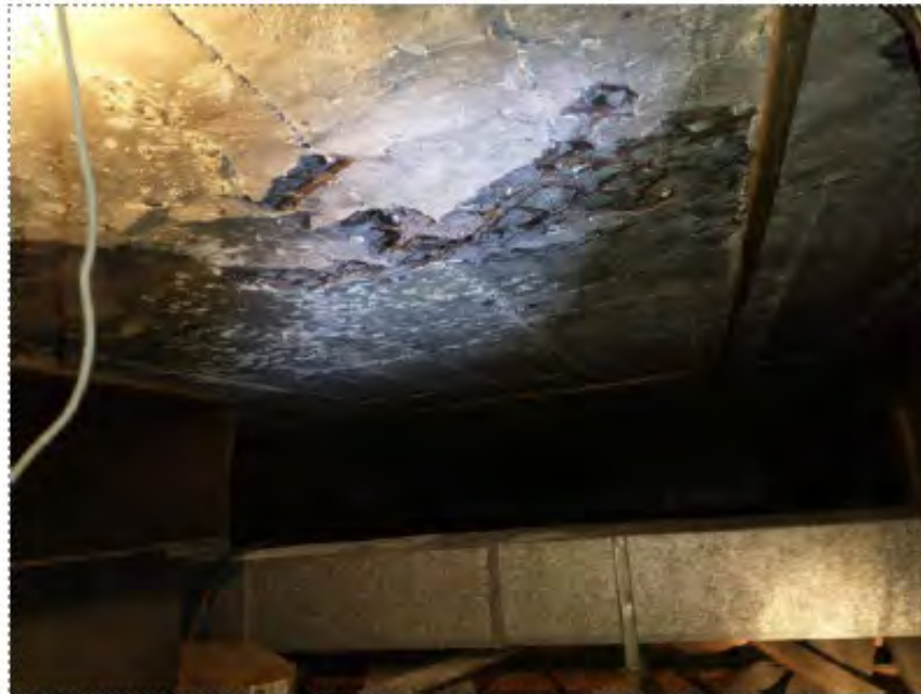
Photo No. 2 – Roof slab over Bar 318.
