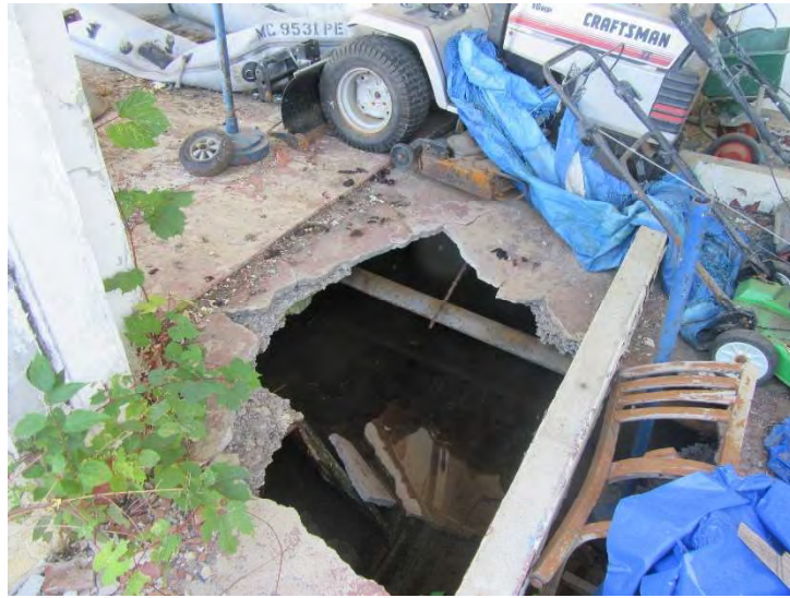
Photo 79 Hole in Pool Deck Below Northeast Terrace 2019
