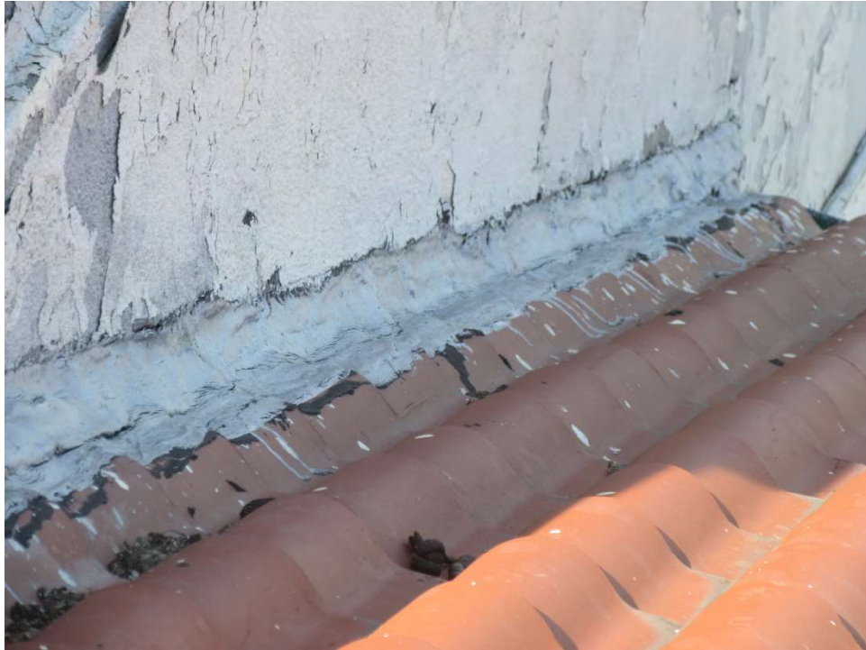
Photo 47 Rake Wall Flashing Buried Under Mastic
