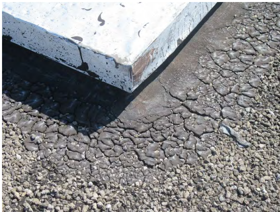
Photo 56 Damaged Flashing
