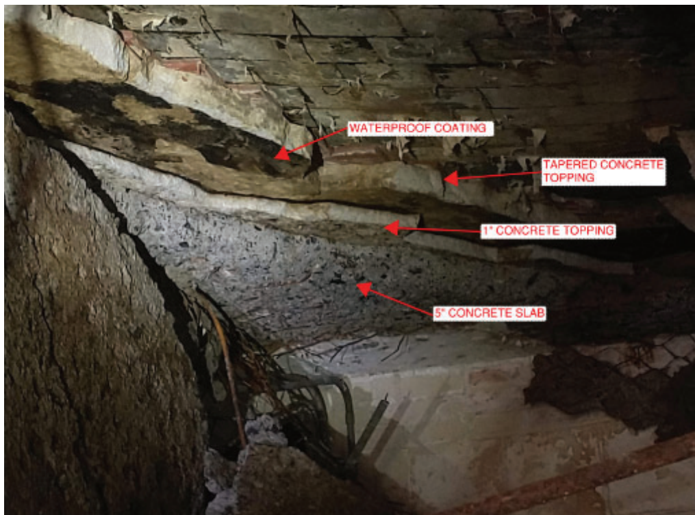
Photo No. 6 – Terrace slab layers.
