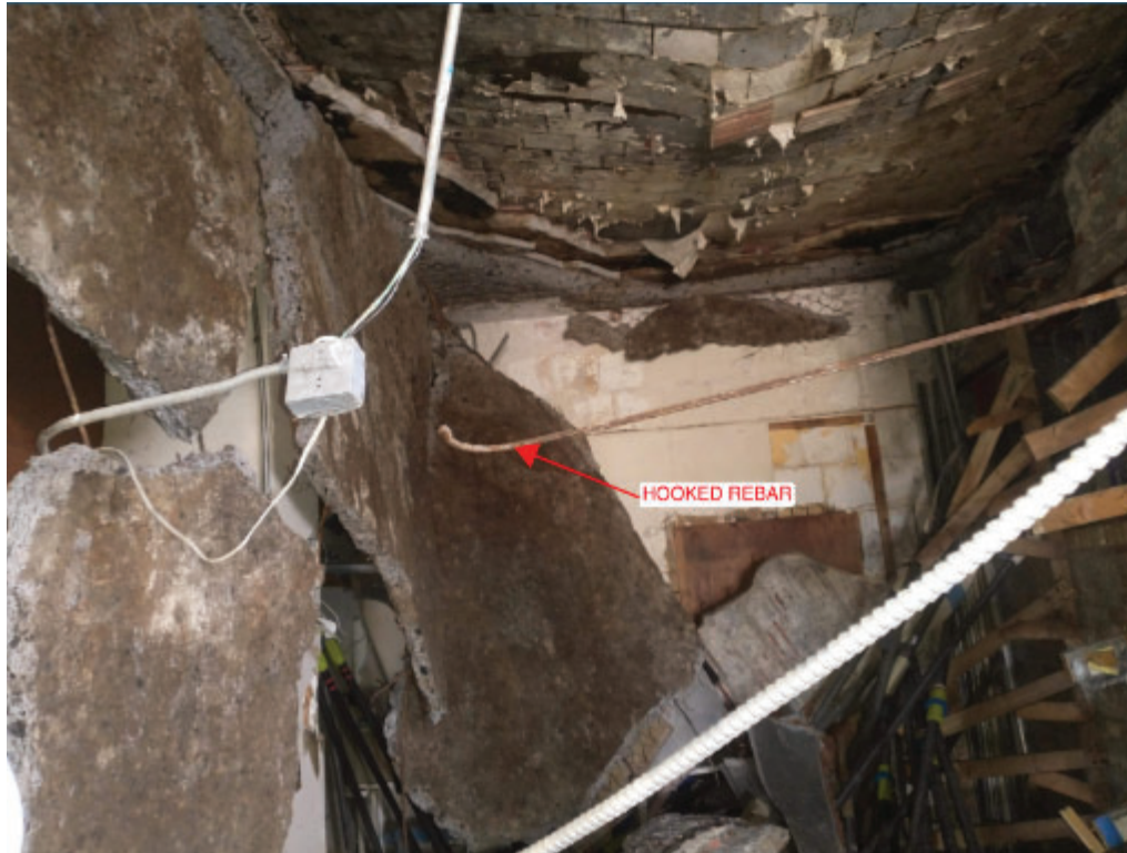
Photo No. 5 – Failed west side terrace slab.
