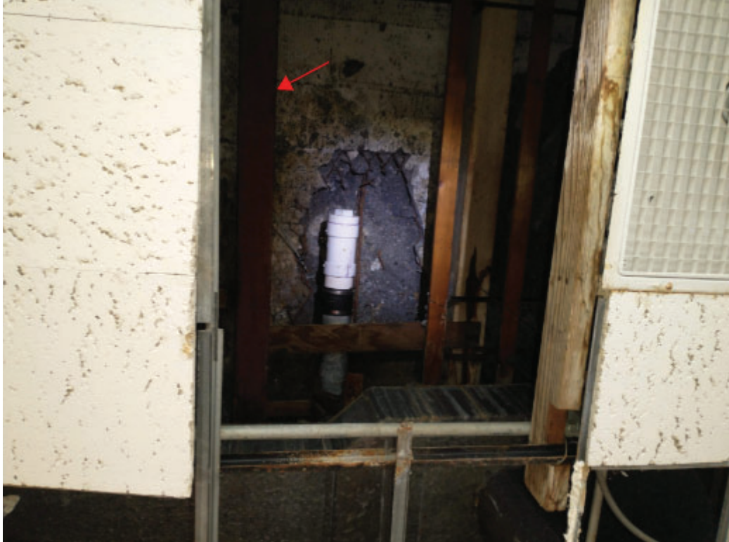
Photo No. 1 – Roof slab above Lounge 319. Rusted reinforcing and spalled concrete. Note newer red steel.
