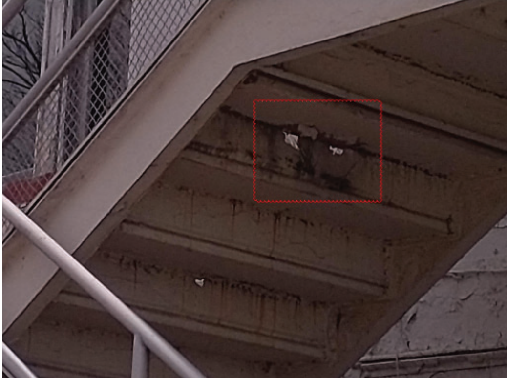
Photo No. 25 – Rusted stair riser.
