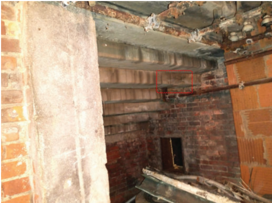
Photo No. 24 – Spalled stone stair riser.
