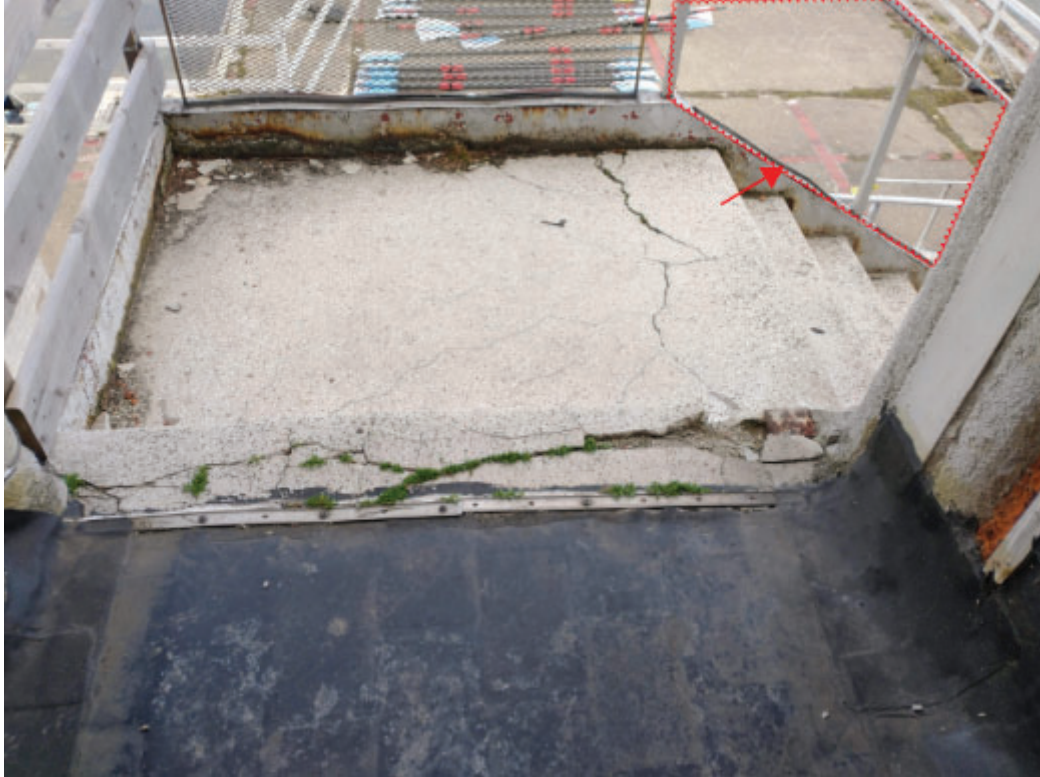
Photo No. 27 – Deteriorated stair landing. Missing rail screen.
