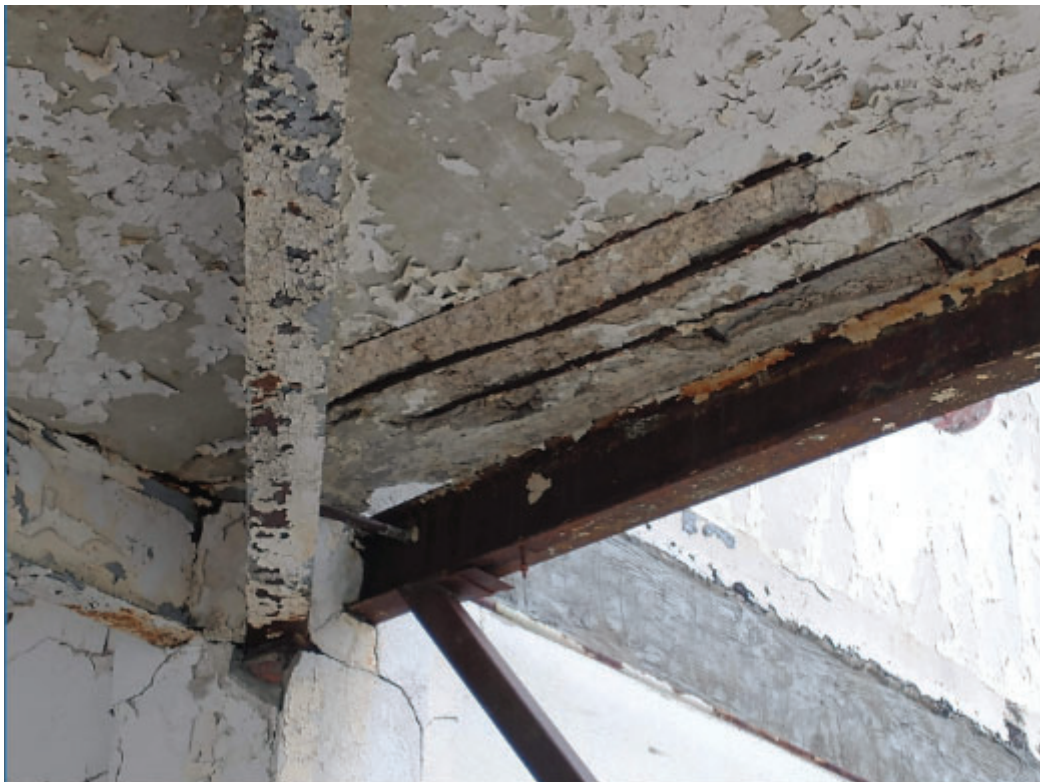
Photo No. 10 – Terrace roof slab with rusted rebar, spalled concrete.
