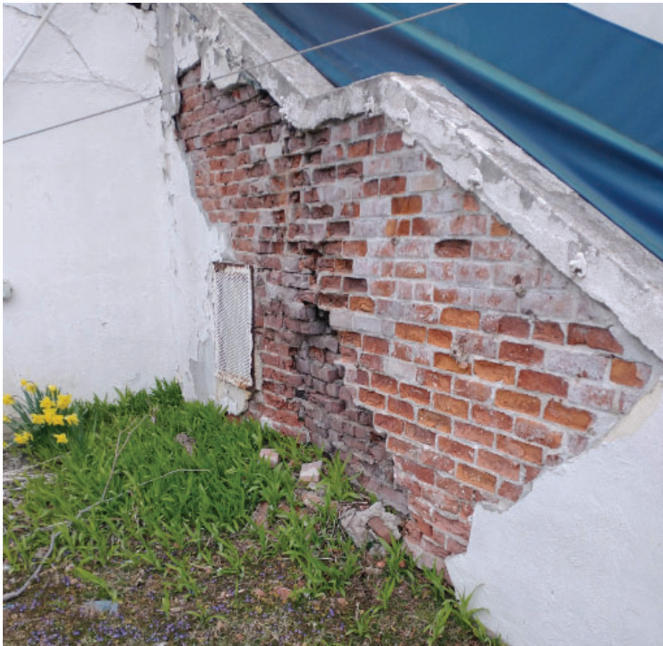
Photo No. 20 – Deteriorated masonry at south main entrance.
