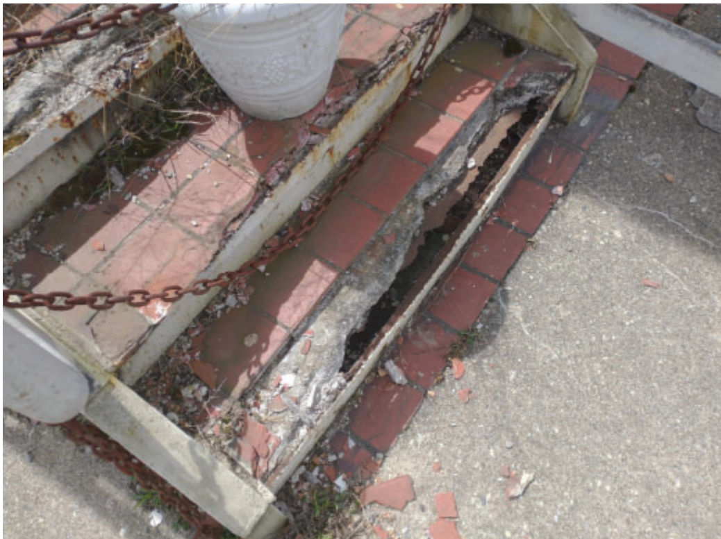
Photo No. 26 – Deteriorated stair riser.
