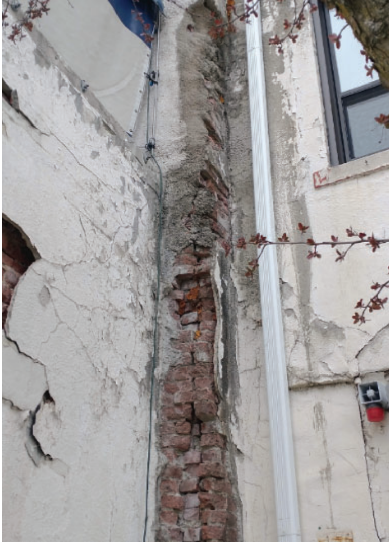
Photo No. 21 – Deteriorated brick masonry near south main entrance.
