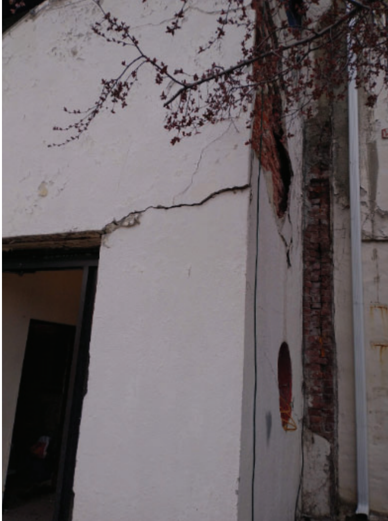
Photo No. 22 – Cracked stucco.
