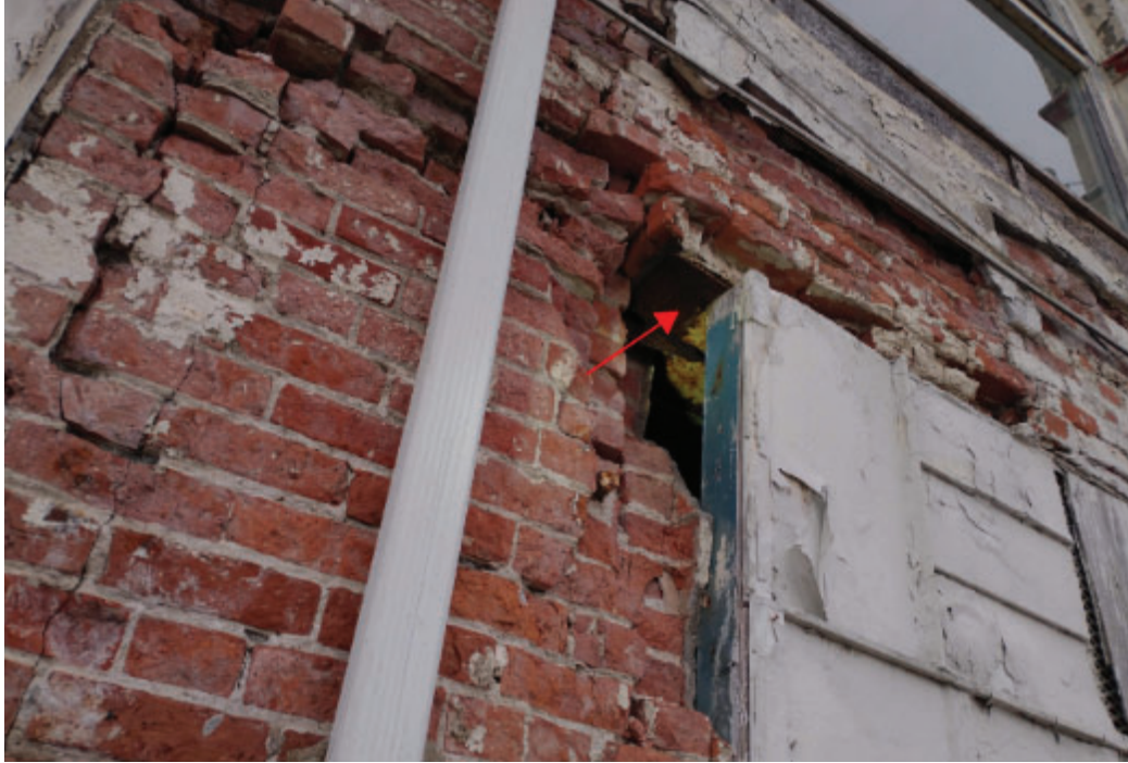
Photo No. 19 – Deteriorated masonry, brick missing at steel bearing.
