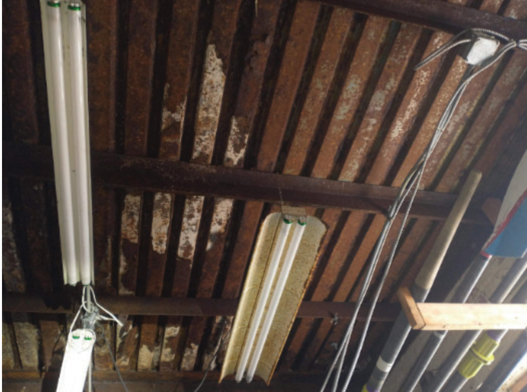
Photo No. 9 – Underside of 1950s replacement slab.
