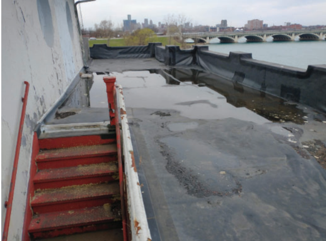
Photo No. 17 – Ponded water at the north terrace, west end.
