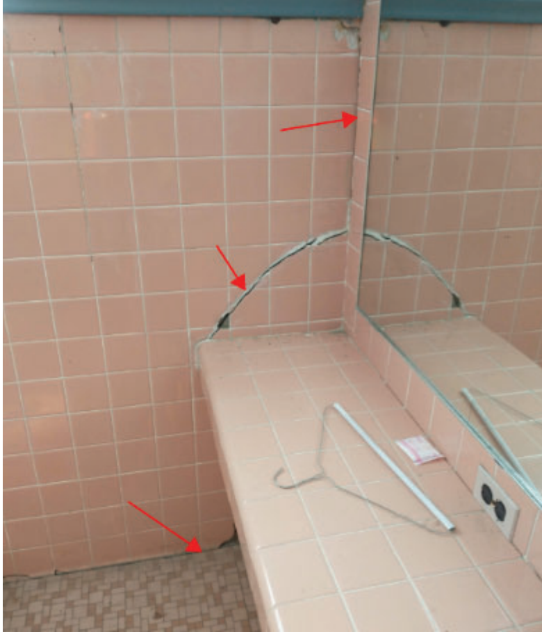
Photo No. 23 – Cracked exterior wall at Women's Locker Room.
