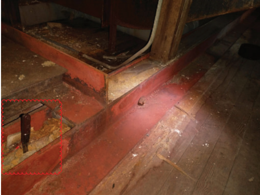
Photo No. 3 – Bottom chord wood truss over Conference Room 309. Red steel reinforcement. Note knife in rotted wood.
