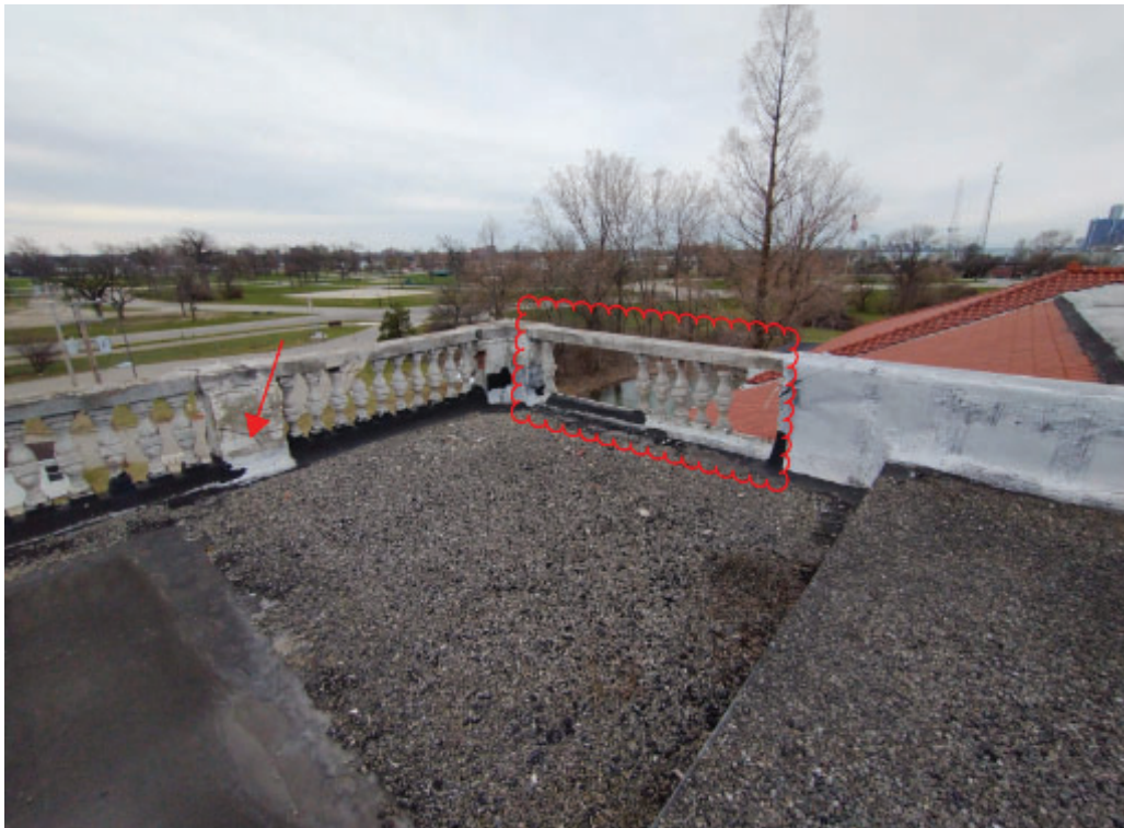
Photo No. 4 – Roof over Lounge 319. Deteriorated railing and posts.
