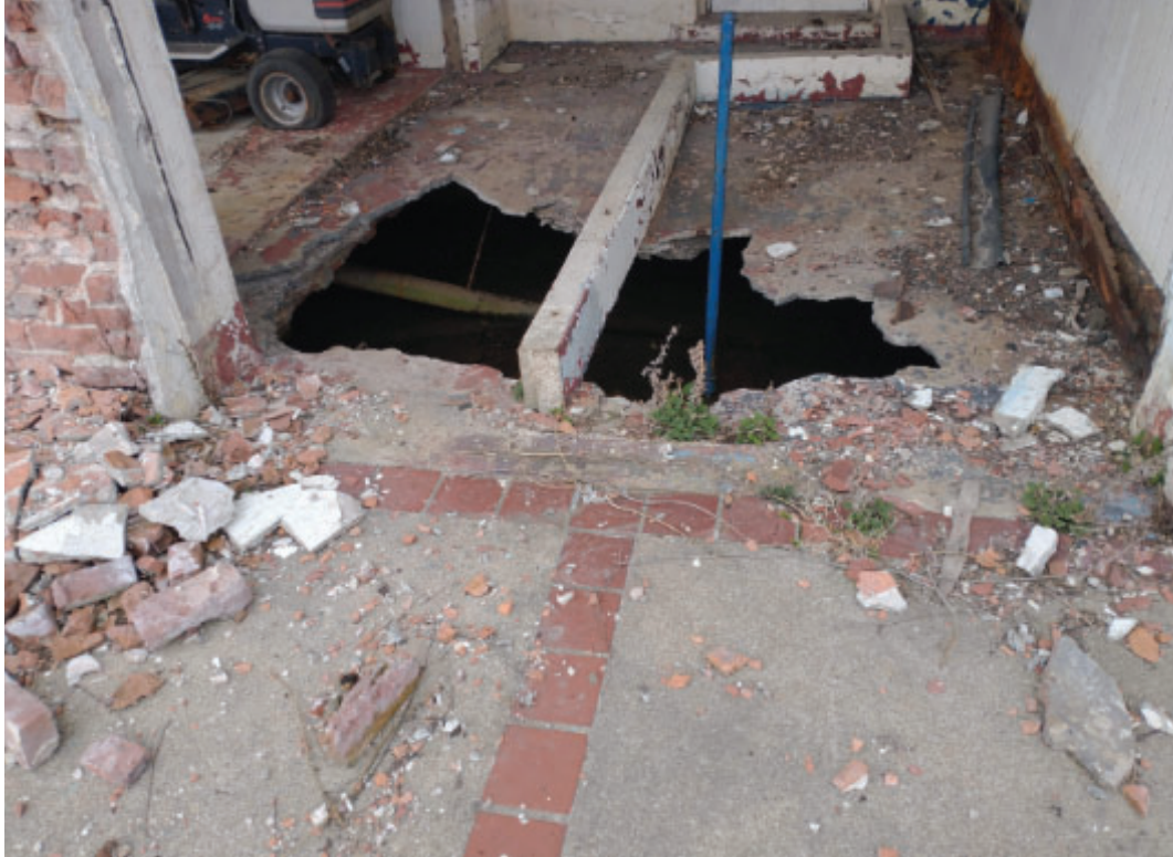
Photo No. 15 – Hole in first floor slab under the north terrace, east end.
