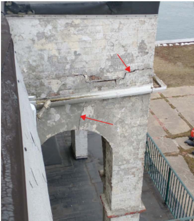
Photo No. 16 – Cracked brick masonry.
