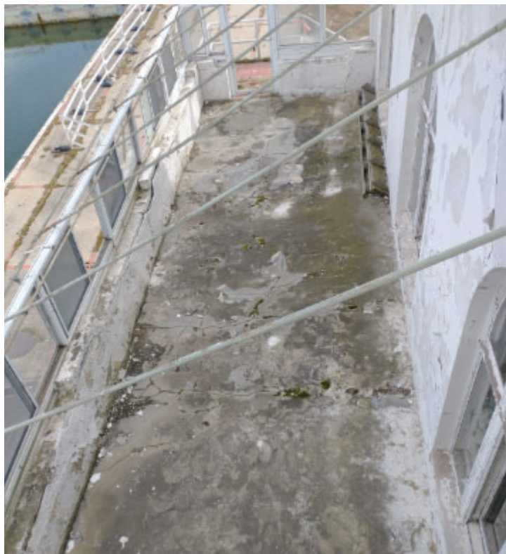
Photo No. 14 – North terrace, east end. Deteriorated concrete topping, loose canopy and screen wall framing.
