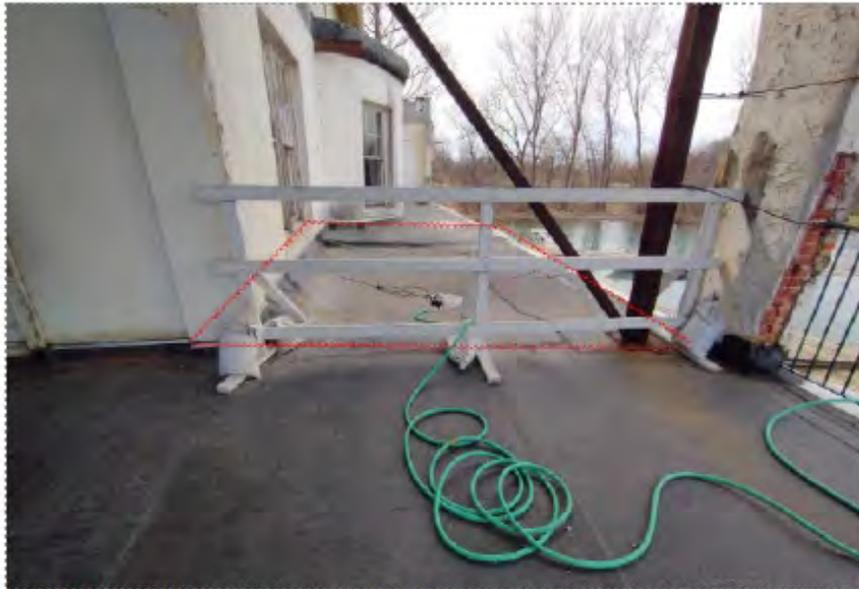
Photo No. 8 – Failed terrace slab viewed from topside.
