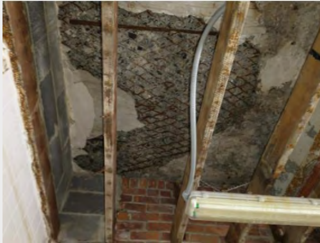
Piece of terrace slab showing rust stain from a rebar and rusted steel mesh
