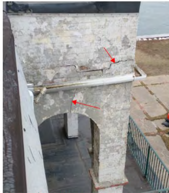
Cracked brick masonry
