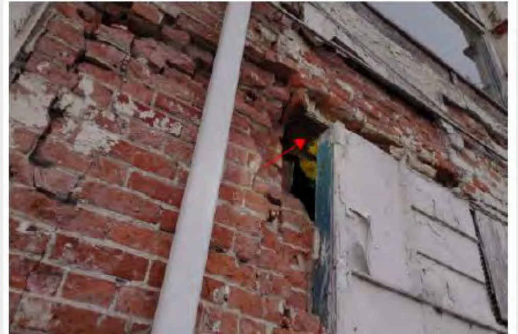
Deteriorated brick masonry, brick missing at steel bearing.
