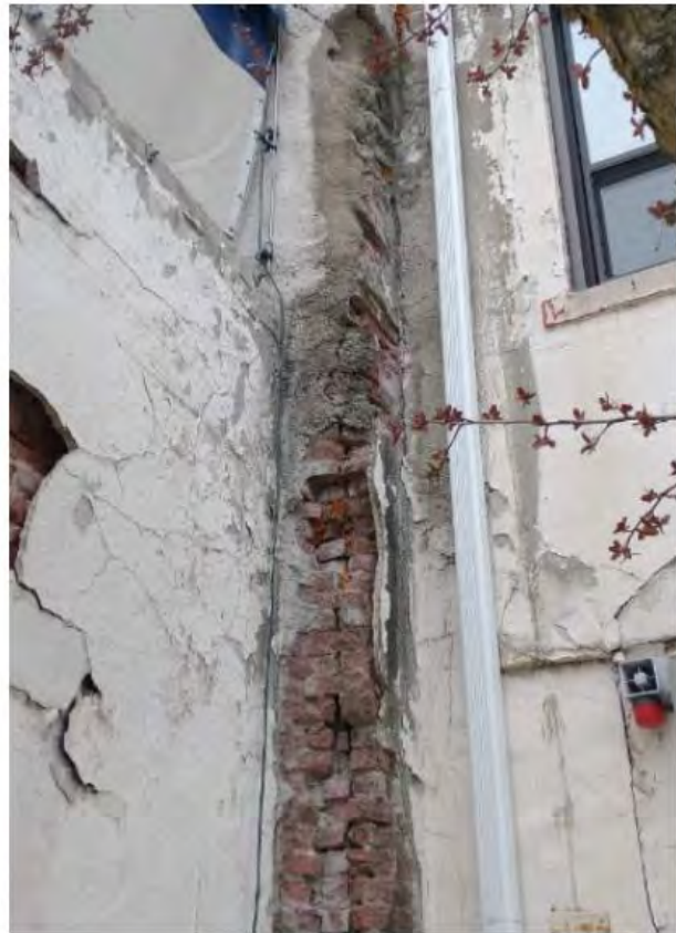
Deteriorated brick masonry near south Main Entrance
