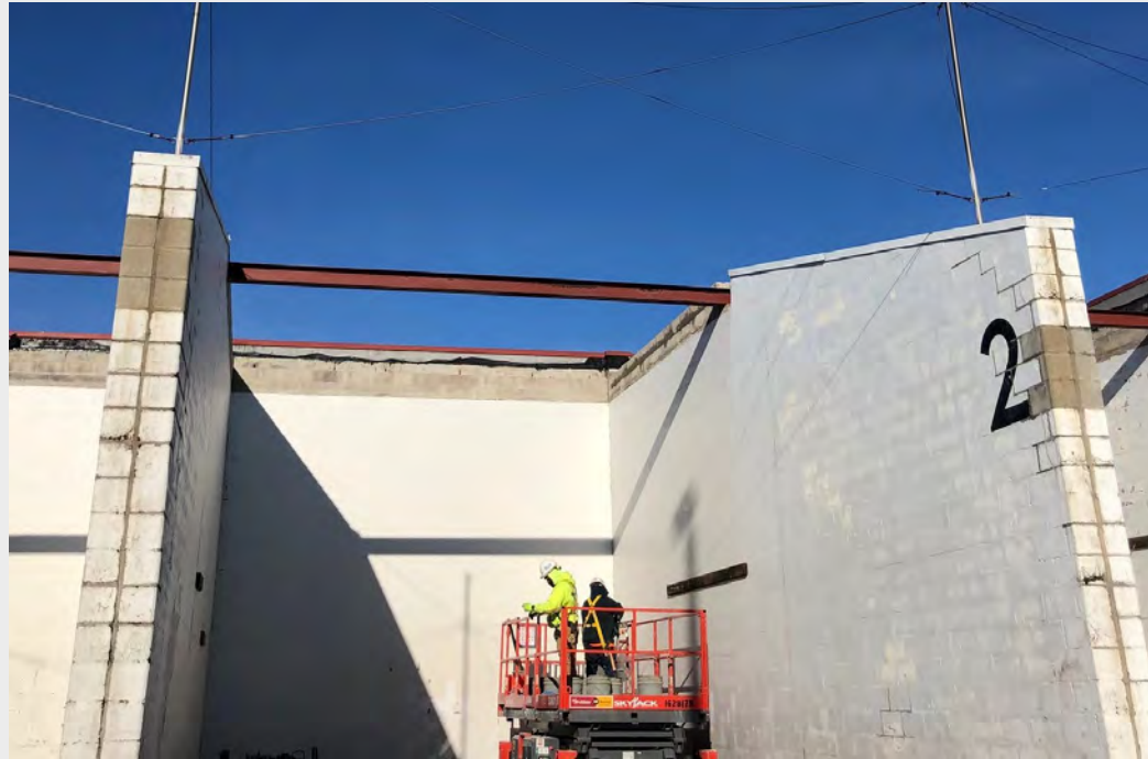
Final scope of work includes masonry repairs, coping installation and painting of walls
