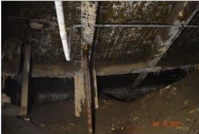
PHOTO NO. 3: Outer pool underside exhibited cracks with efflorescence staining, stalactites and active water ingress.
