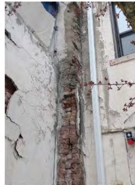
Photo No. 21 – Deteriorated brick masonry near south main entrance.
