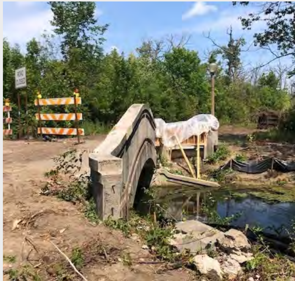
MDOT scope includes concrete repair of historic Bridge, embankment stabilization and decking maintenance.
