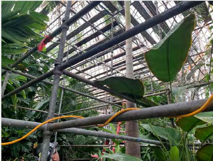
Scaffolding being erected around plants and planter walls.
