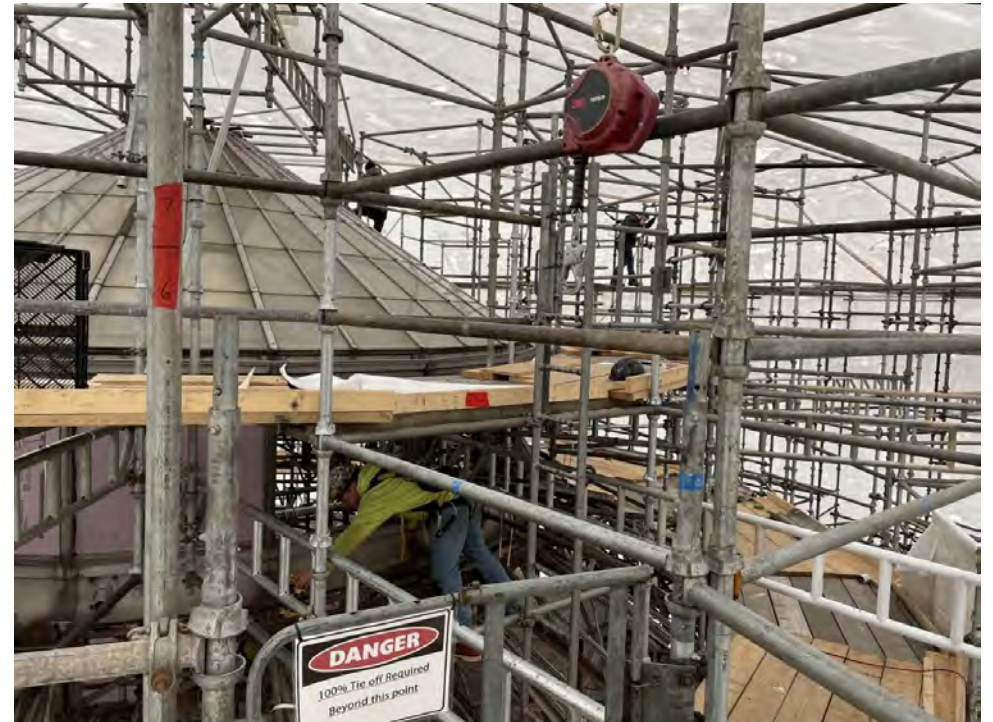
Interior of dome wrapping, glass removal underway
