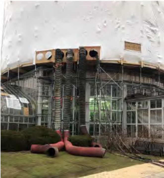
Ventilation hoses to bag house for hazardous material containment
