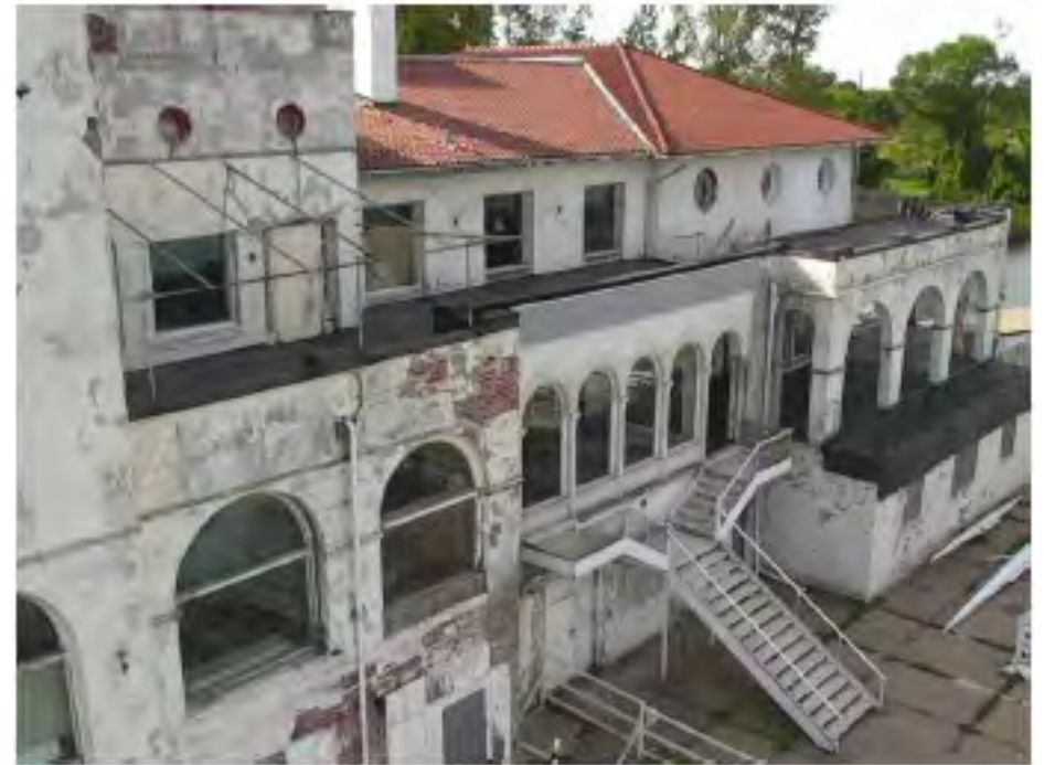
North side of the building compromised by water filtration over the years
