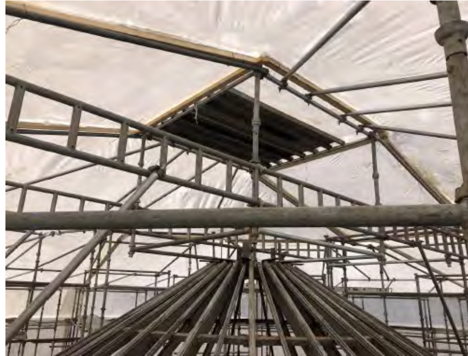
Sub contractor has had to make several repairs to wrapping due to high winds and snow loads
