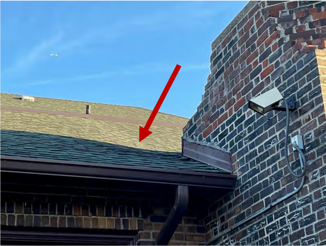
Structural issue apparent in roof dip
