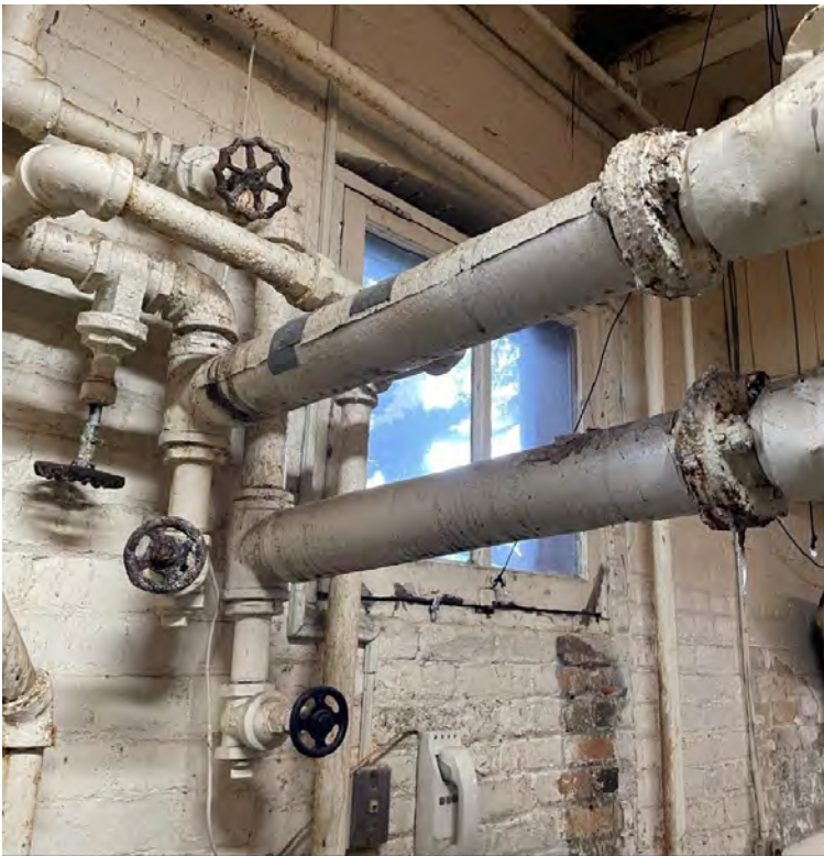
Boiler lines require repairs, and new valves on lines and radiators
