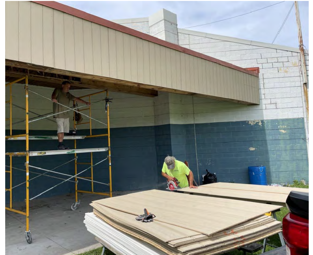
New fascia panels installed 8/16/2023
