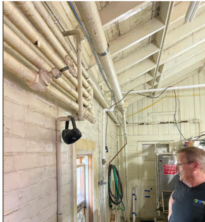
Boiler lines require repairs, and new valves on lines and radiators
