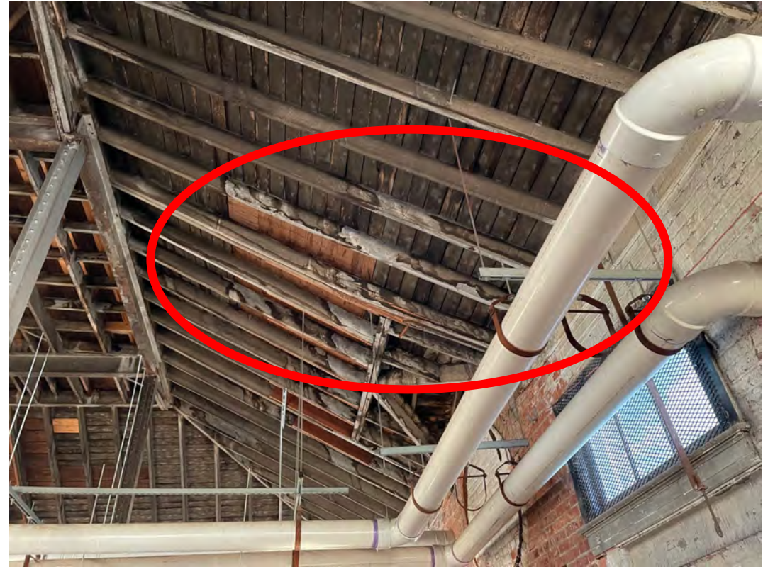
Roof is under- supported and needs replacement and reinforcement to stabilize roof.
