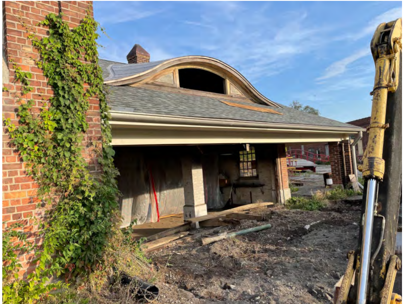
Boarded panels removed and concrete excavation
