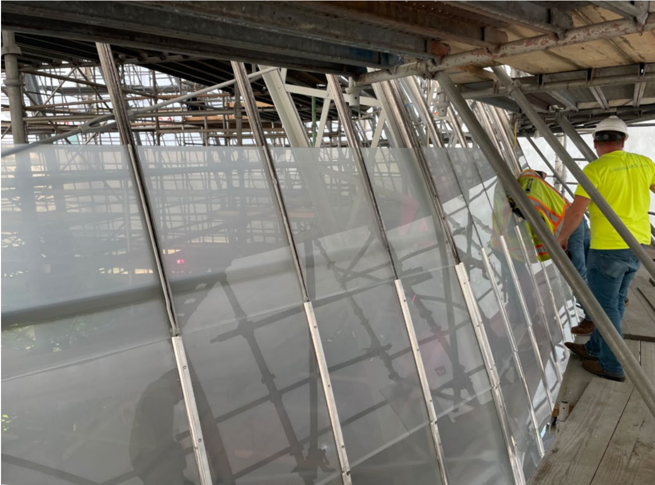
New glass installation in upper dome
