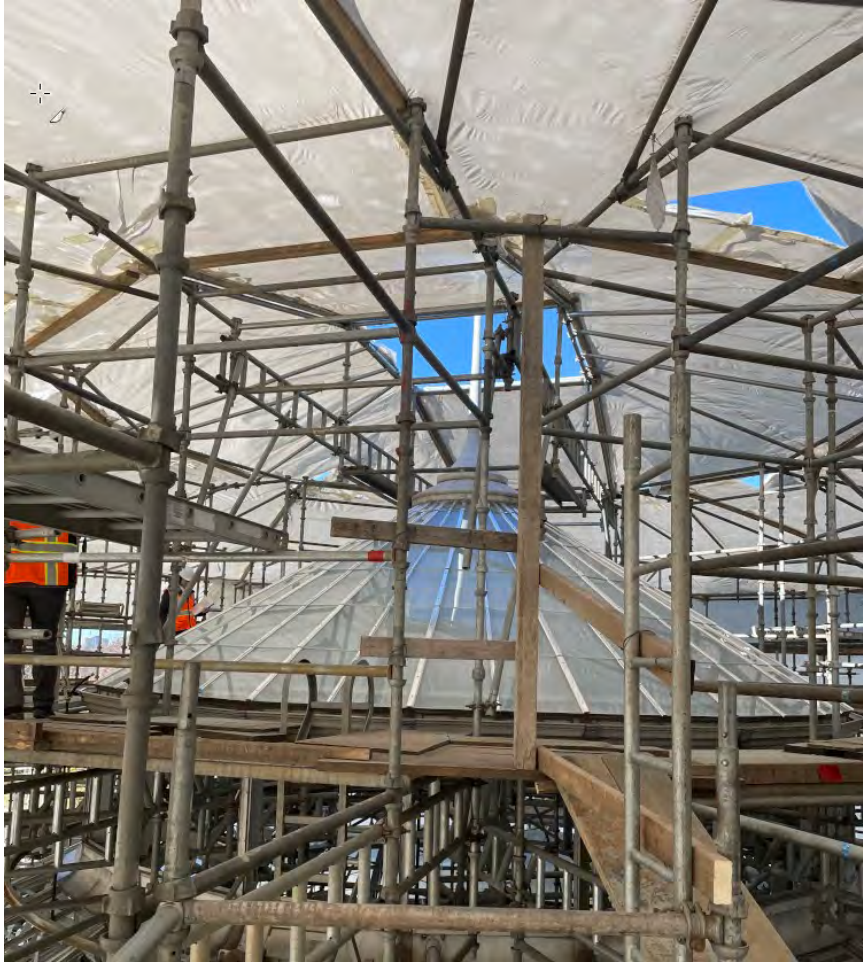
New glass installation in upper dome
