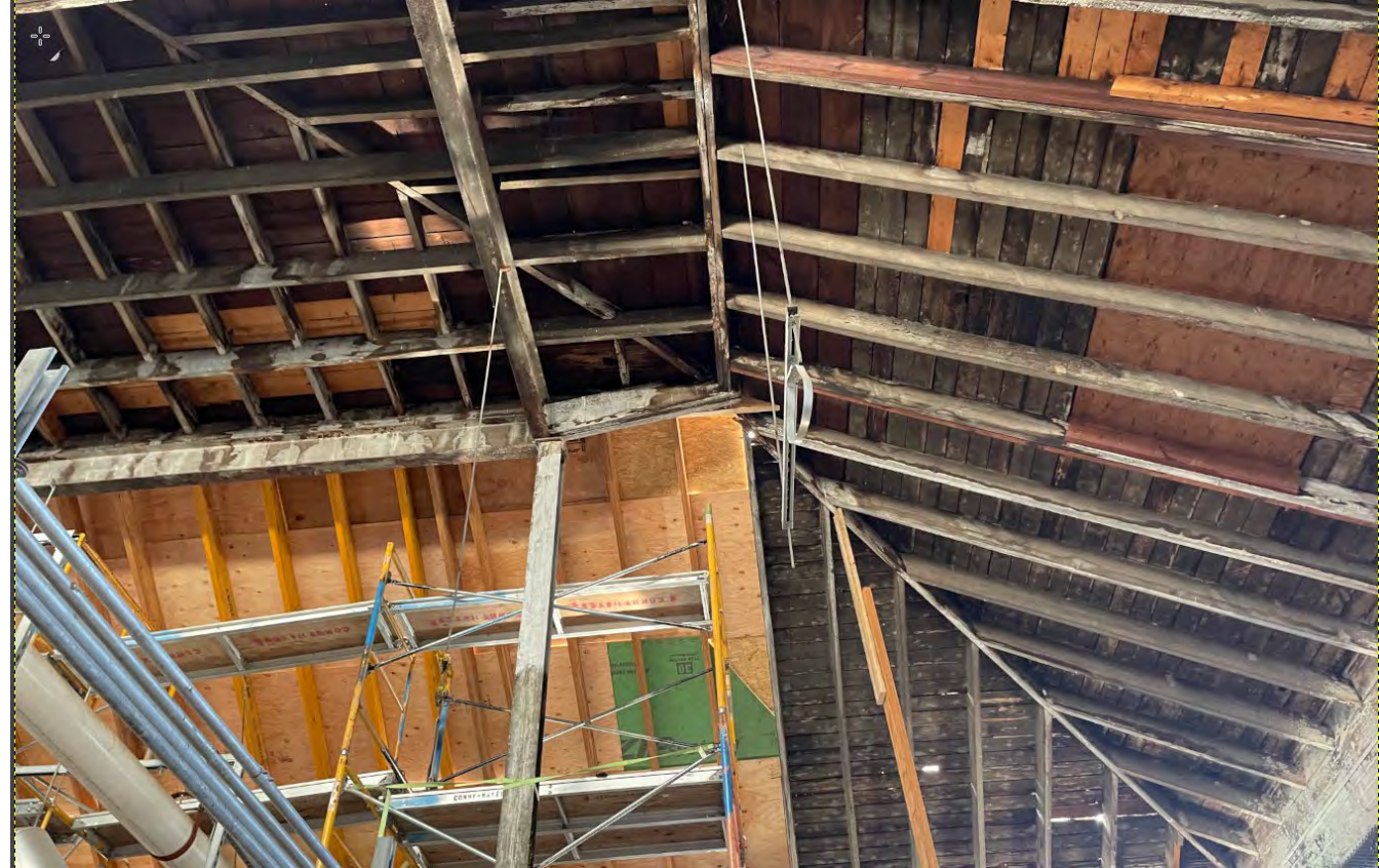
Roof is under- supported and needs replacement and reinforcement to stabilize roof.
