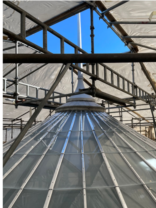
Scaffolding will be removed once glass replacement complete.
