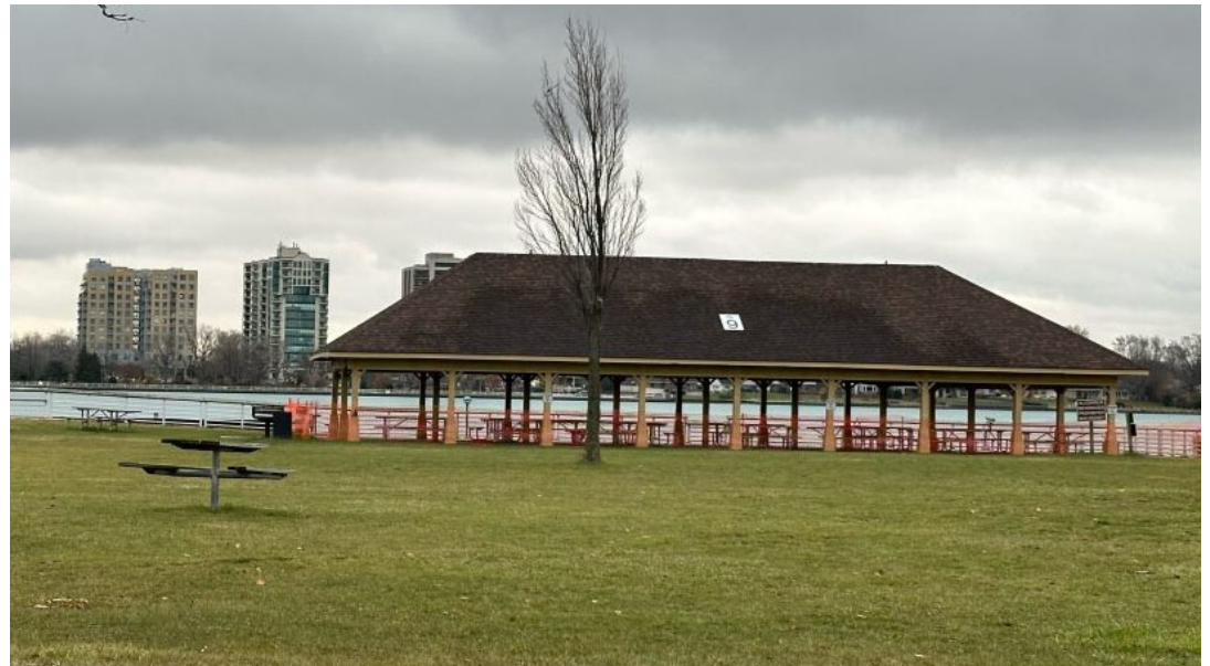
Shelter #9 – closed to the public for repairs
