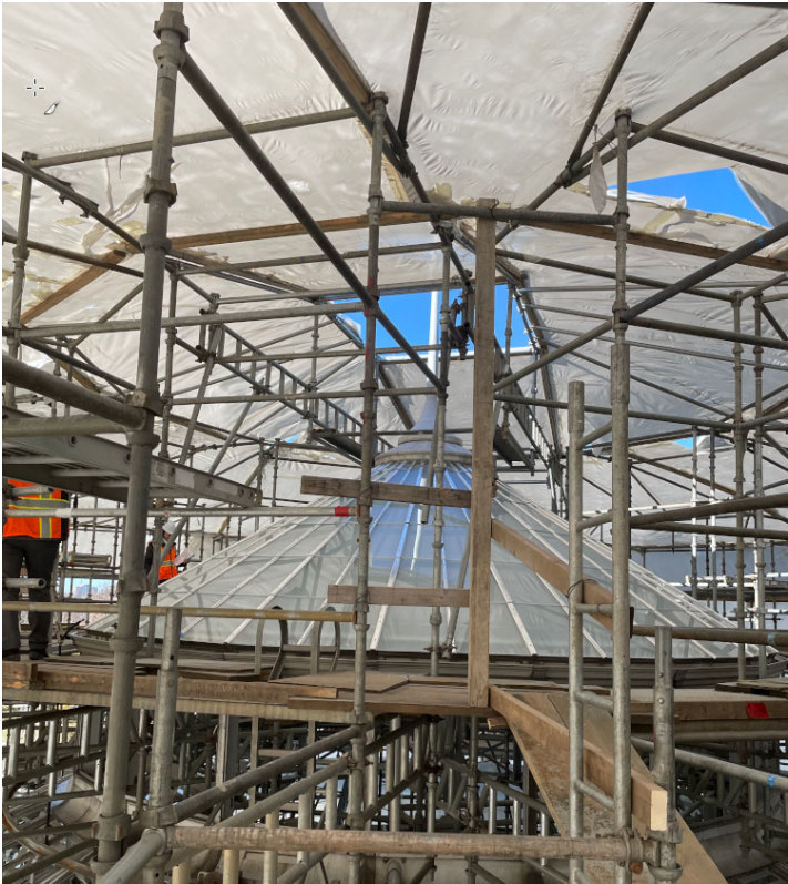
New glass installation in upper dome
