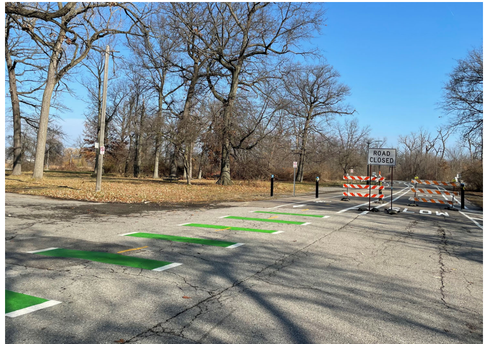
Gate will be installed on Central Ave. in the Flatwoods.
