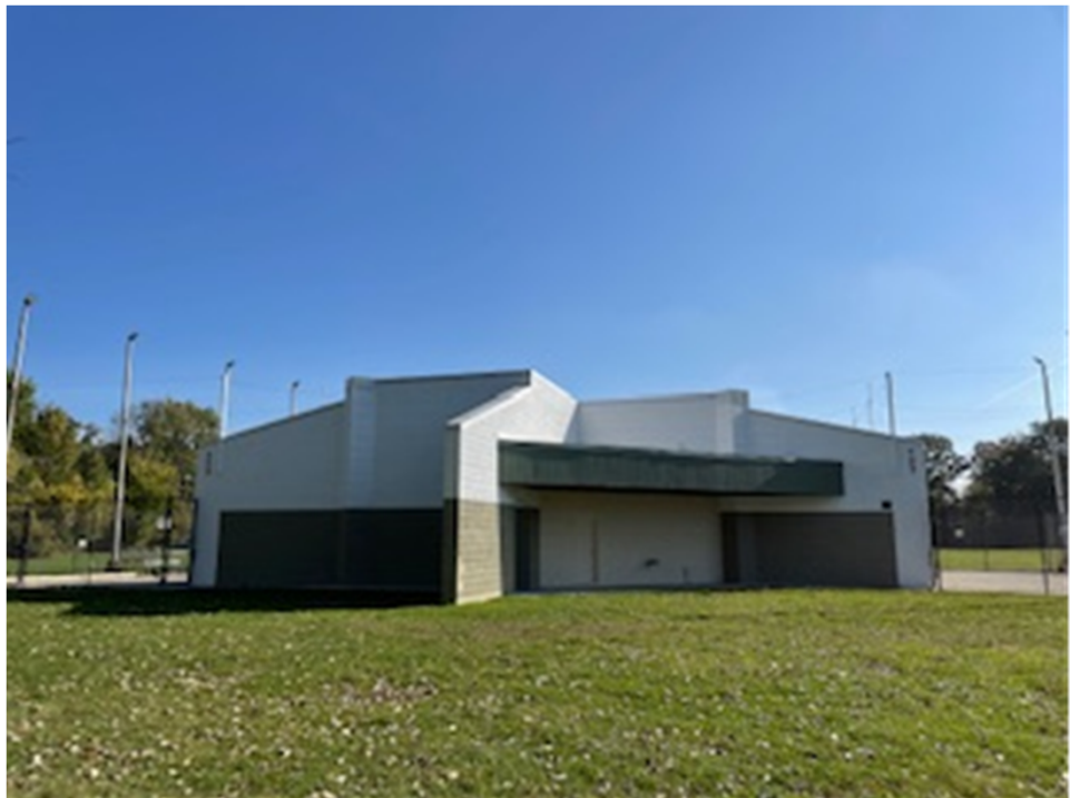
Handball courts stabilized
