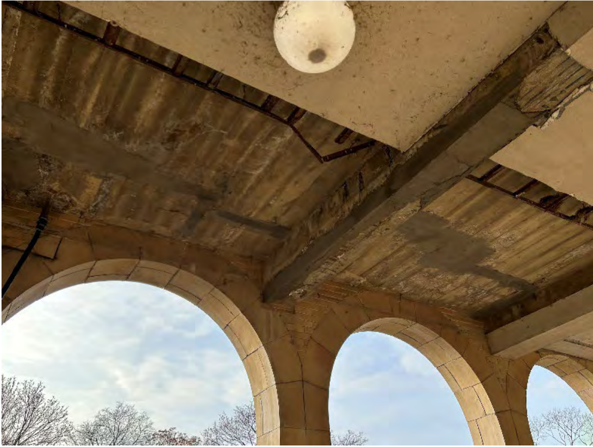
Structural repairs and patching completed
