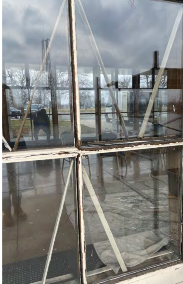
Single glass panes to be replaced with insulated glass
