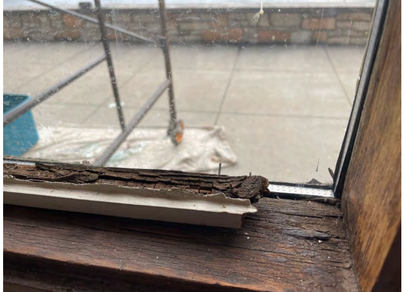
Window framing replacement is being custom made on site.
