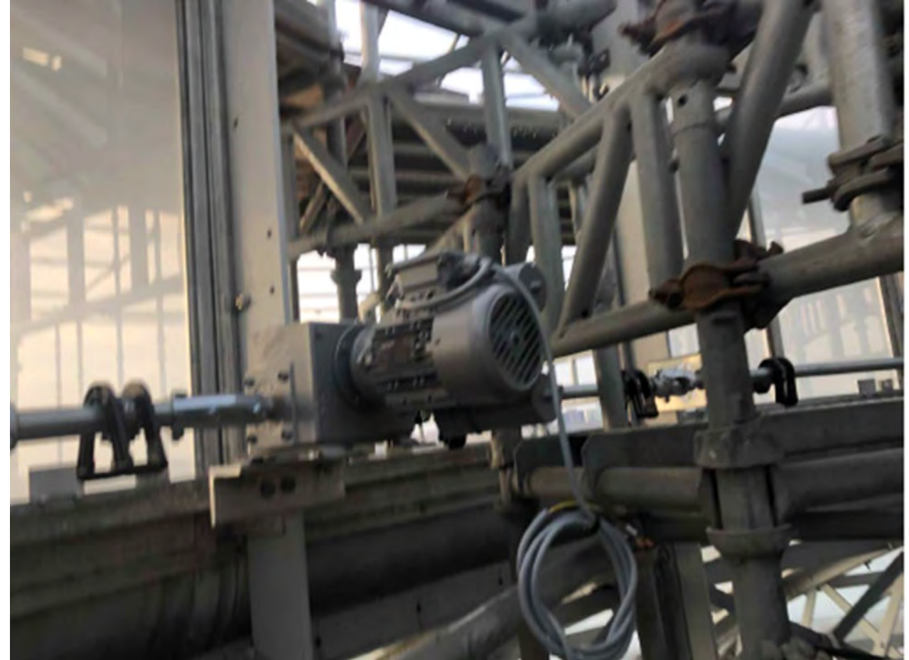
Rack and pinions being installed being installed .
