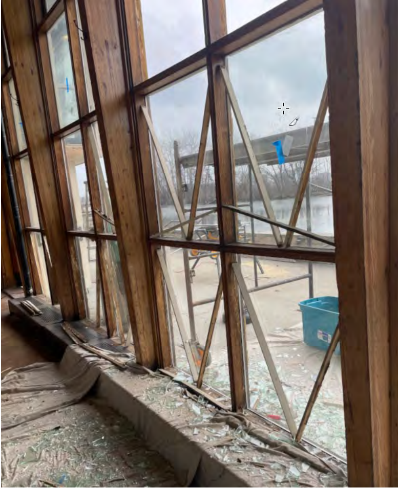
Rotted window framing is being replaced
