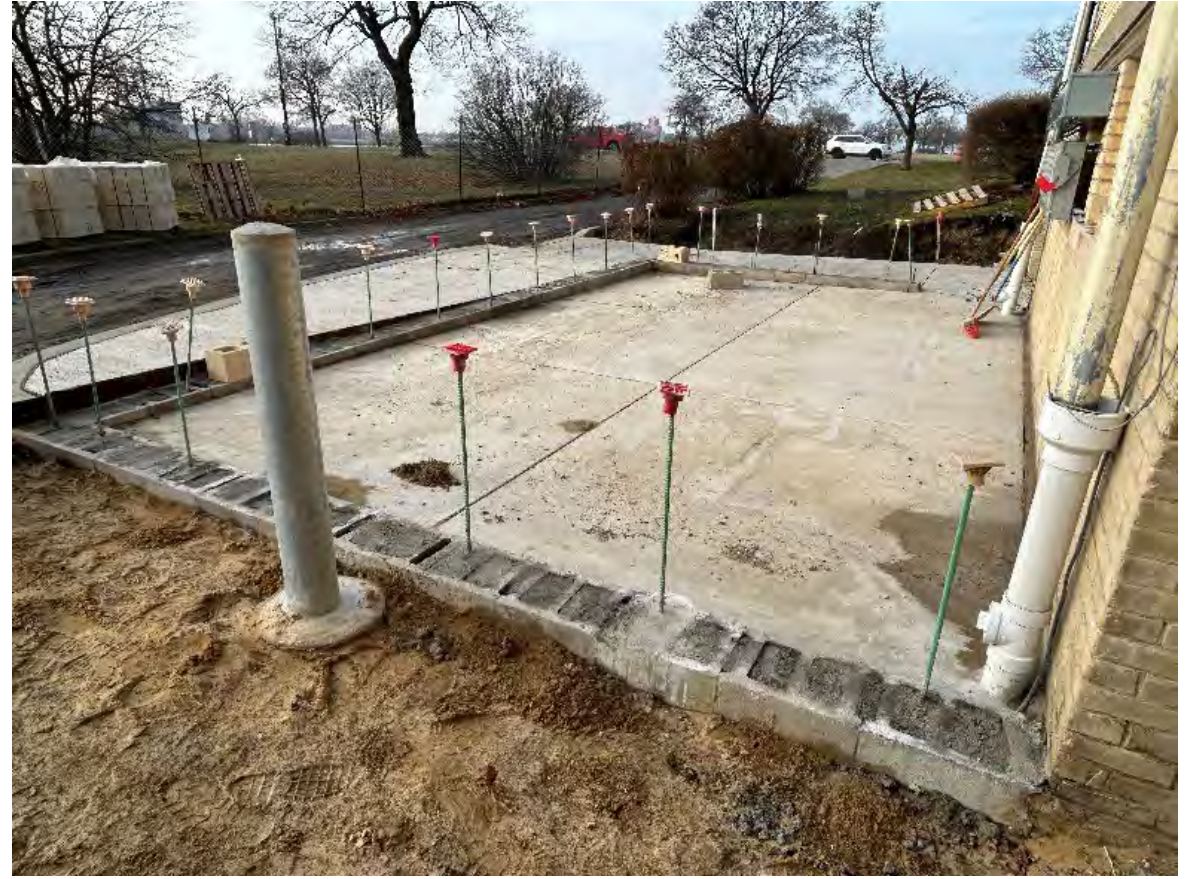
Grouted block base course for new screen wall
