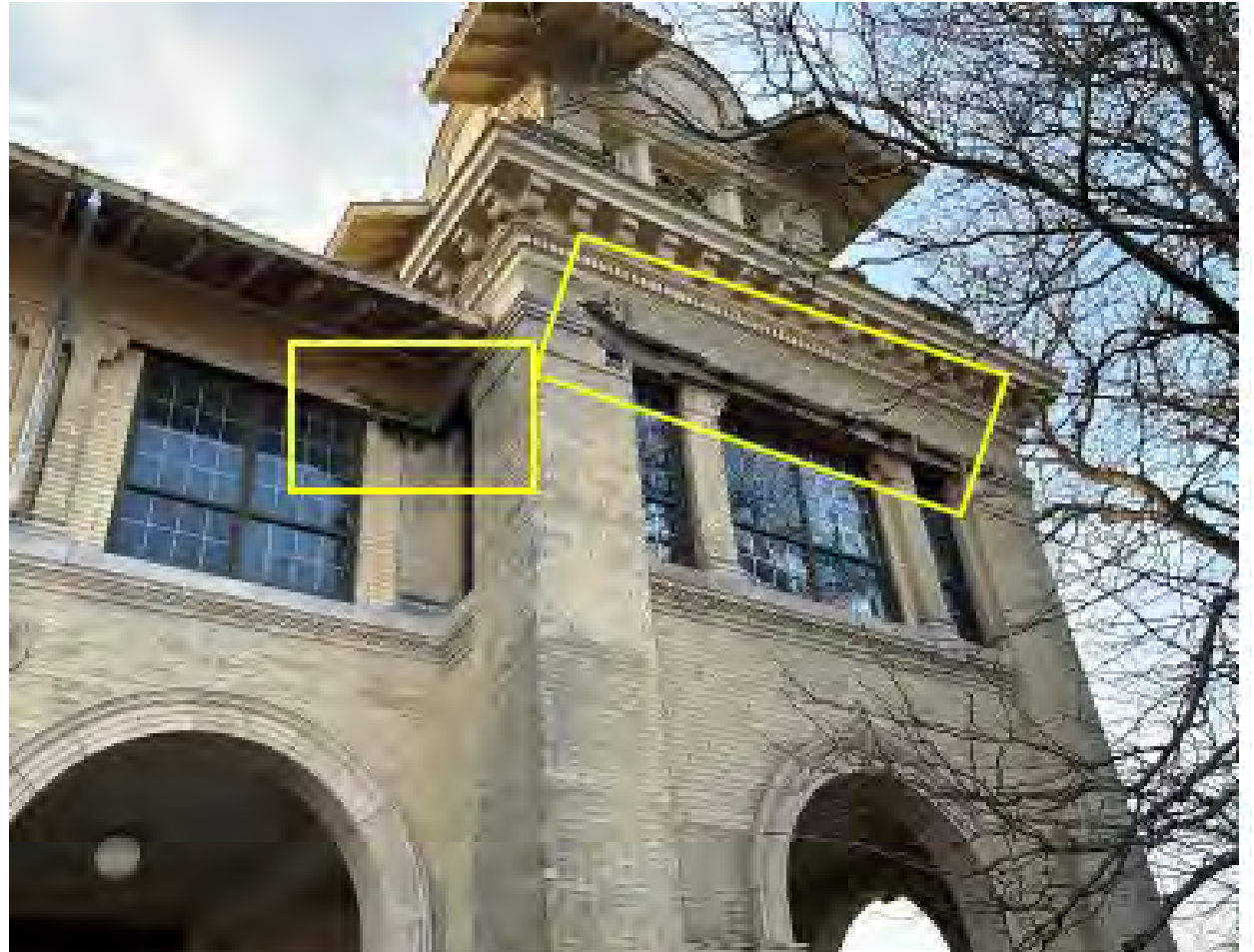
Window steel repairs and replacement, & masonry repairs.
