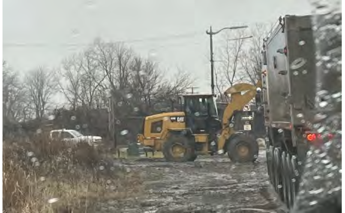
Contractor regrading Staging area to original elevations
