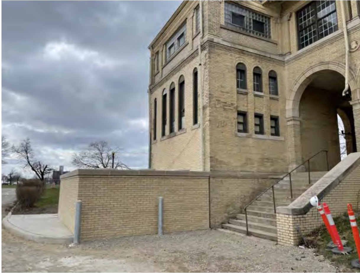
Screen wall for new equipment..
