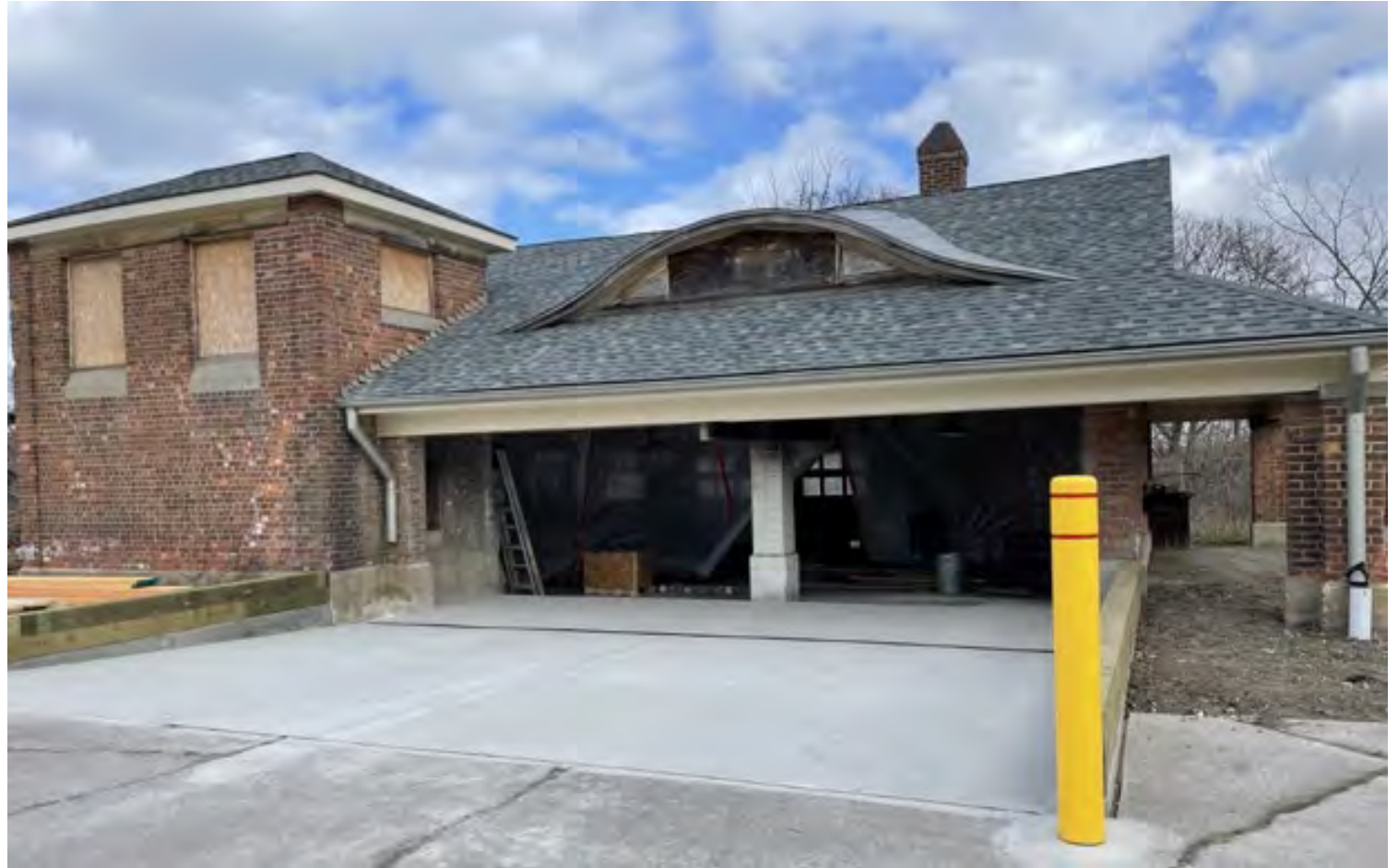
Concrete sloped access and retaining walls complete.
