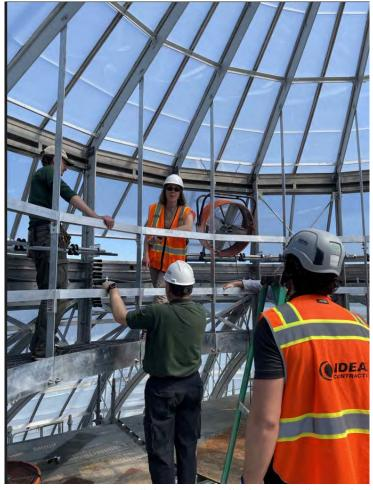
Replacement catwalk being installed at top of cupola – at 80'
