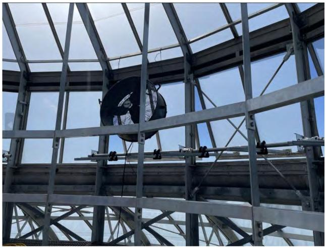
New motors on upper cupola windows and handrails for new upper catwalk
