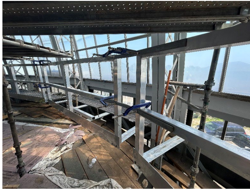
Design of plates between floor grating is being reviewed to complete upper catwalk.
