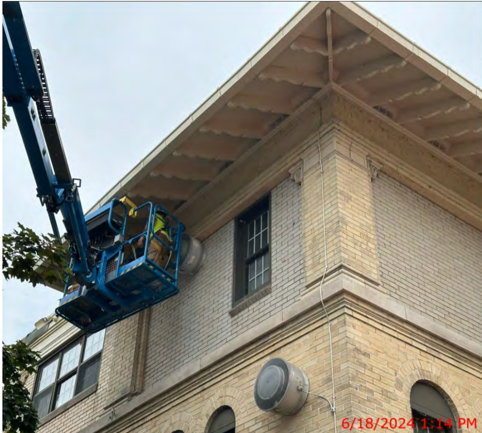
Construction crew working on gutters.
