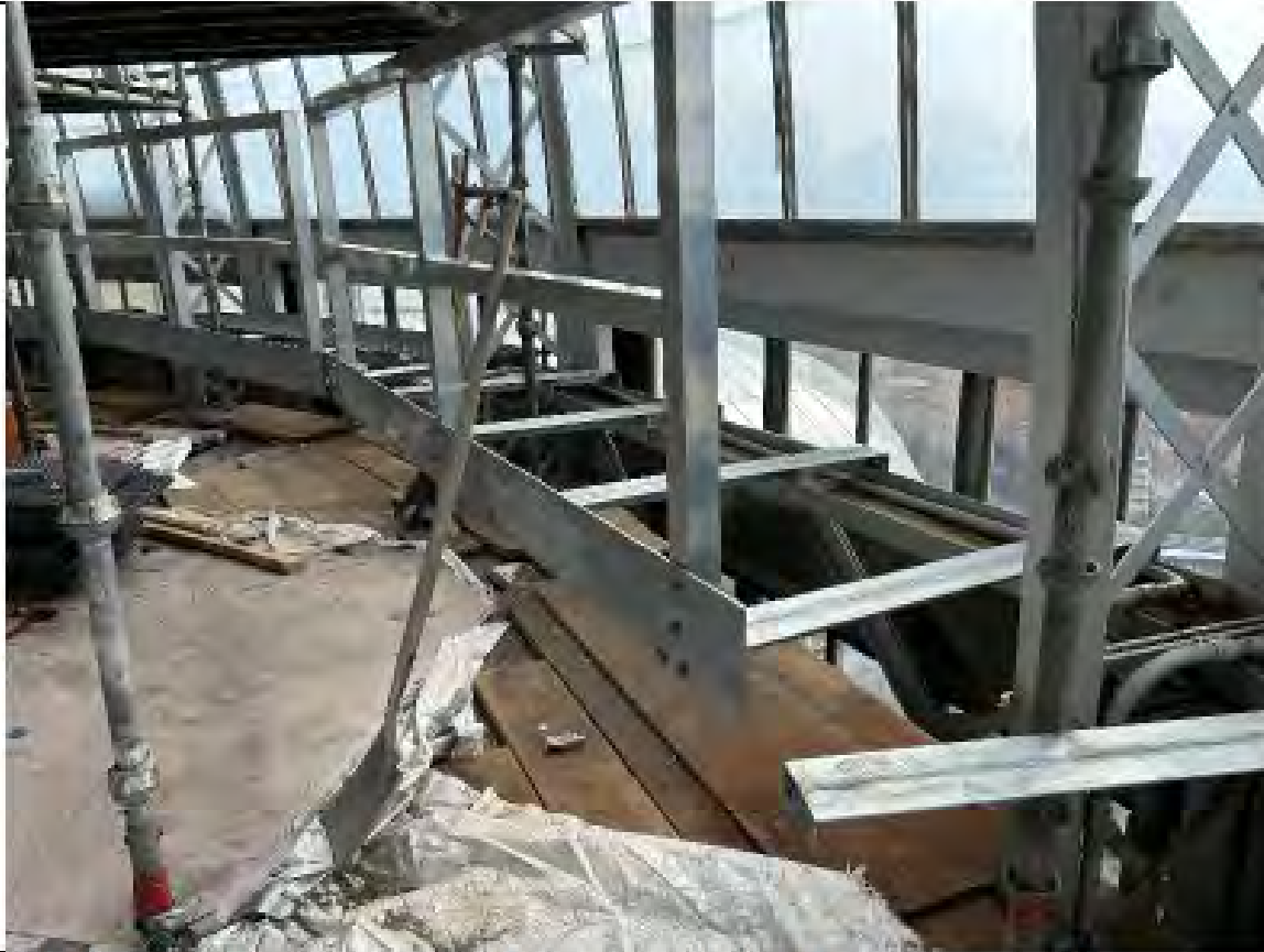
01) View of the floor and railing supports for the lower catwalk area
