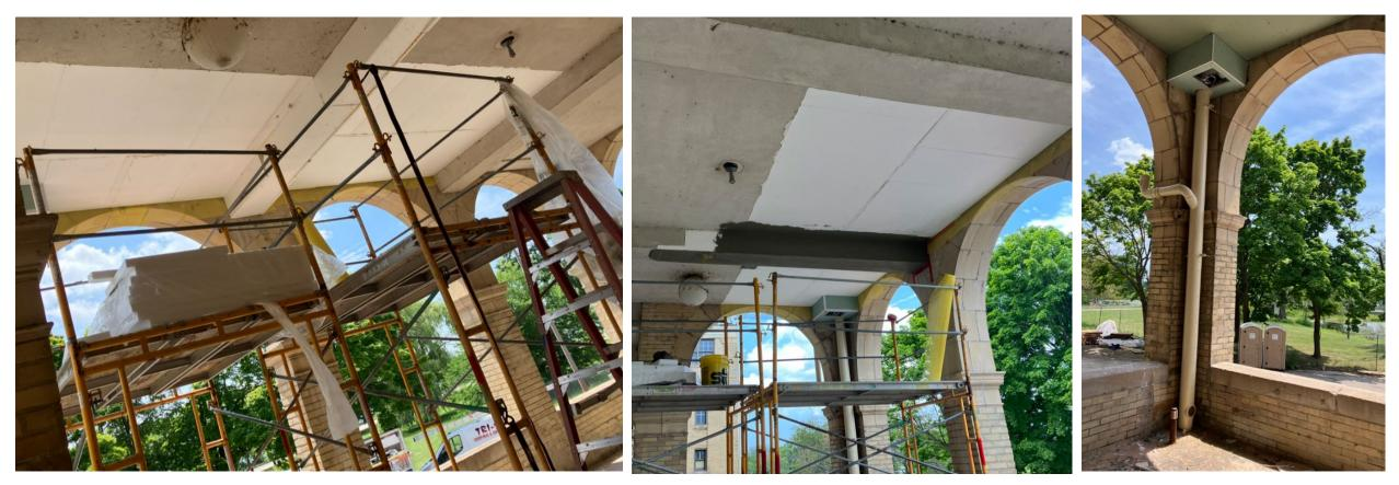
Porch ceiling repairs underway. Damage due to leaks from mechanical room
