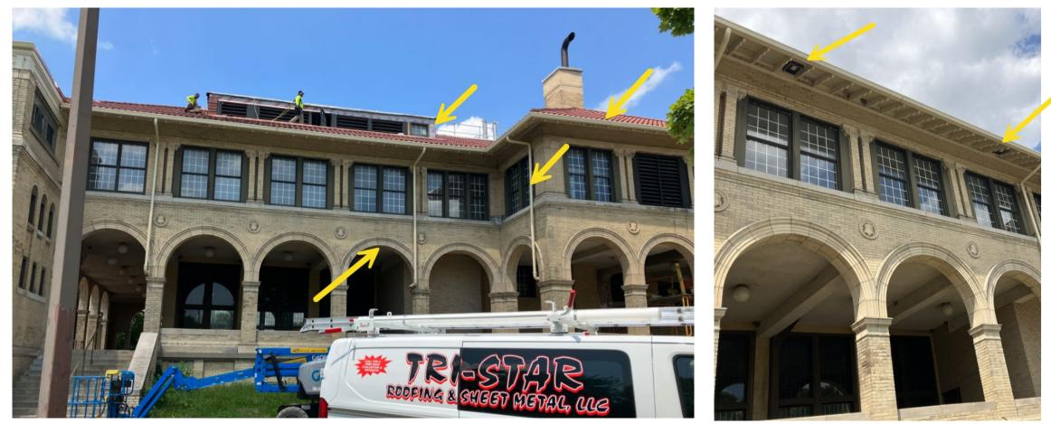
Casino roof, dormer siding, gutters, downspout replacement progressing.
