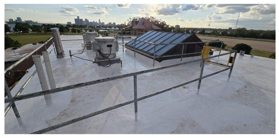
New skylight, security railing and flat roof replacement.
