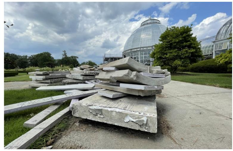
Limestone panels from vestibule will be replaced. Material to be stockpiled for future use within facility.
