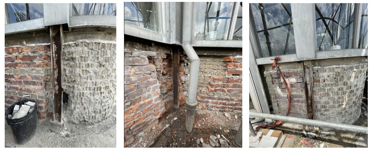
Contractor removing brick around steel supports in preparation of repair/replacement.
