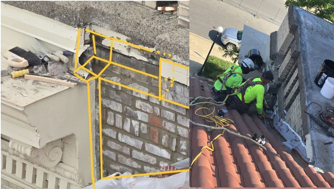
Casino roof, masonry repair and copper flashing installation underway.
