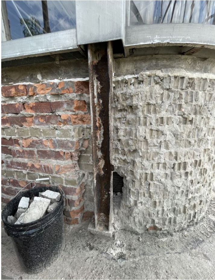
Contractor removing brick around steel supports in preparation of repair/replacement.
