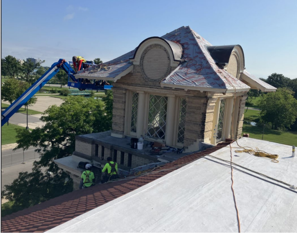
Clay roof tiles installed on towers.
