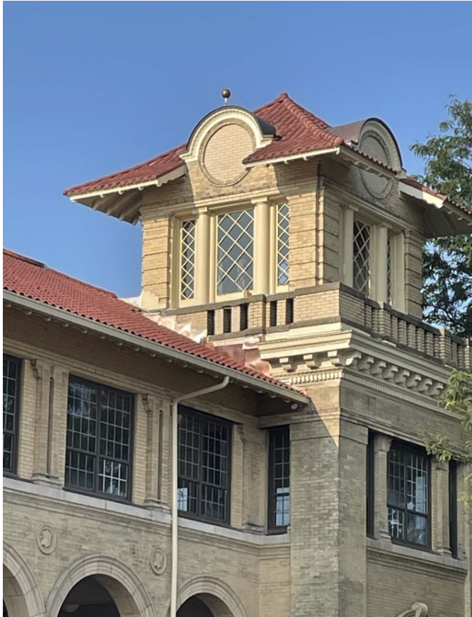
Copper ornament acting as lighting protection placed on towers.
