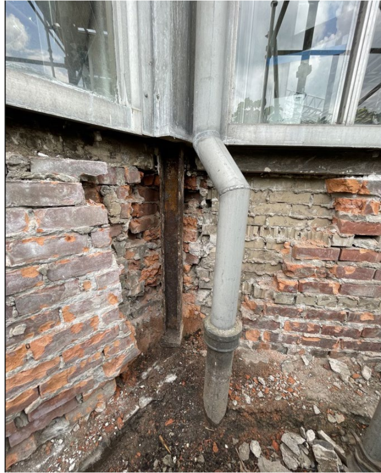
Contractor removing brick around steel supports in preparation of repair/replacement.
