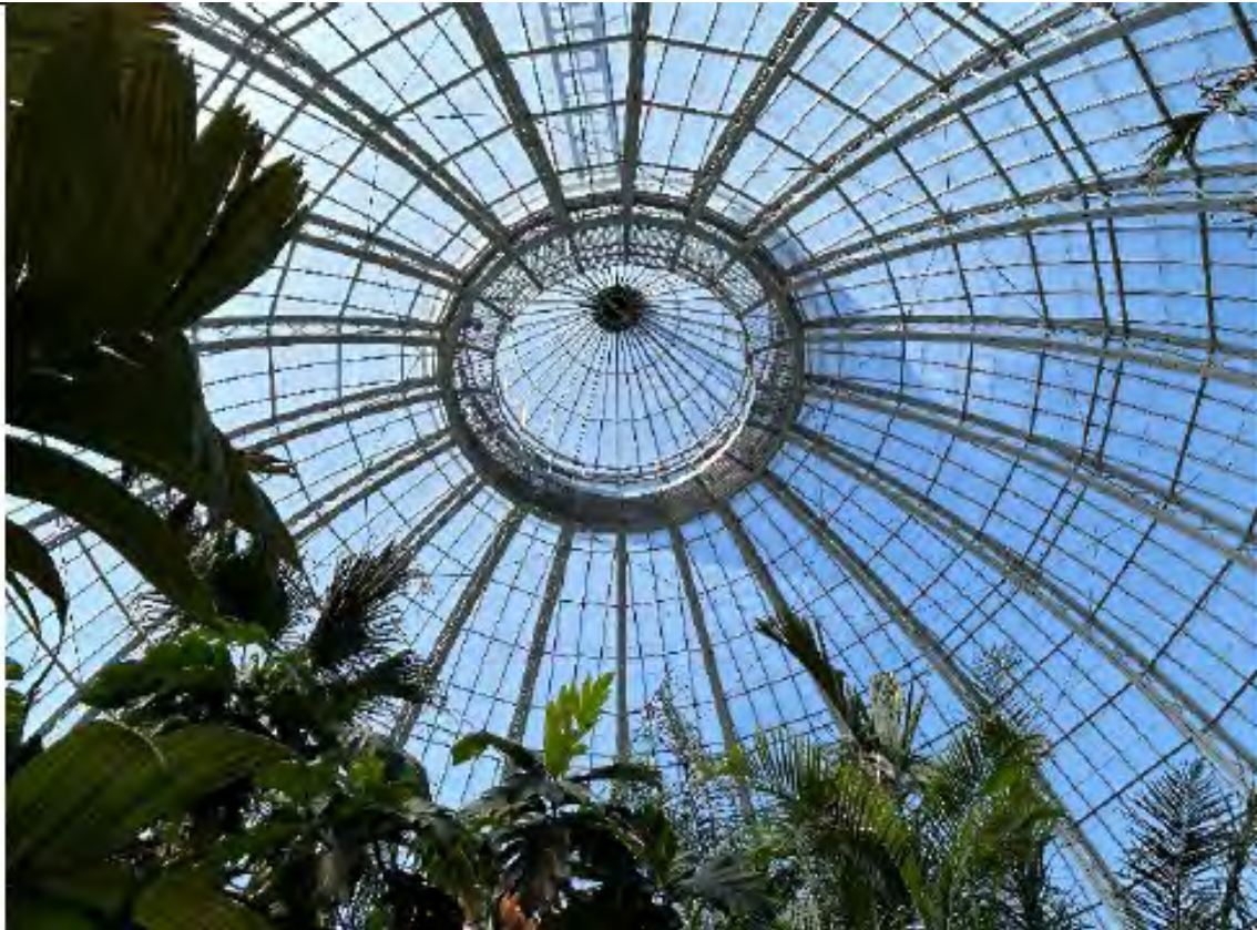
Scaffolding removed on Palm House. New upper catwalk.
