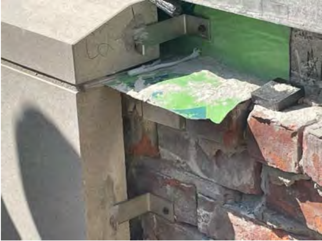
Waterproofing and fastener details for new limestone.
