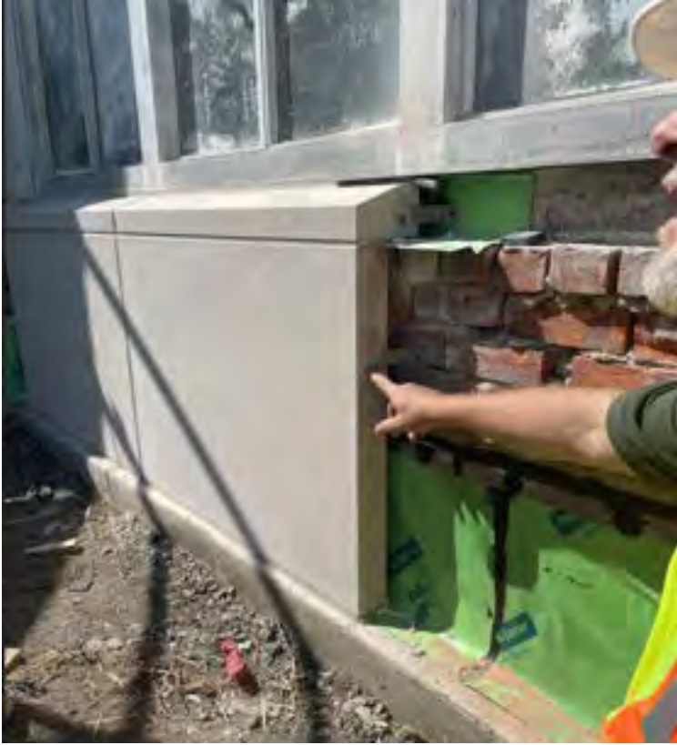
New limestone panels mock-up installed around dome base.
