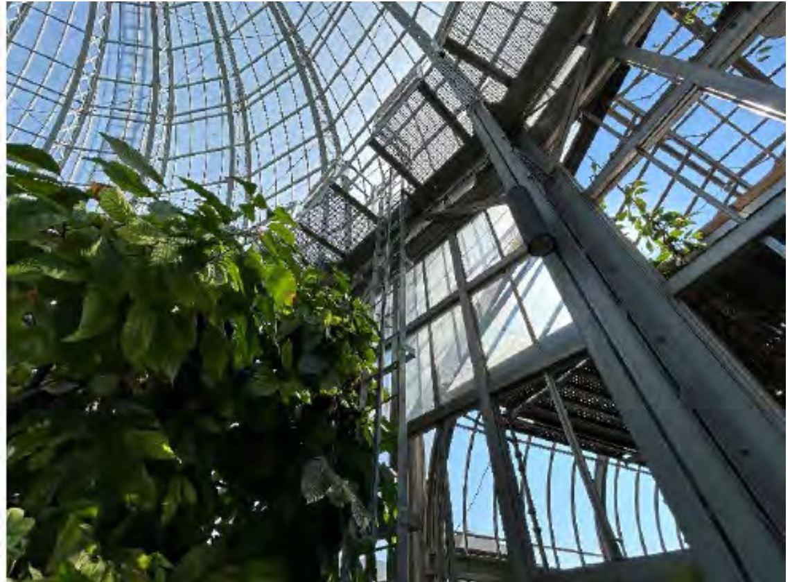
New lower catwalk and safety ladder.
