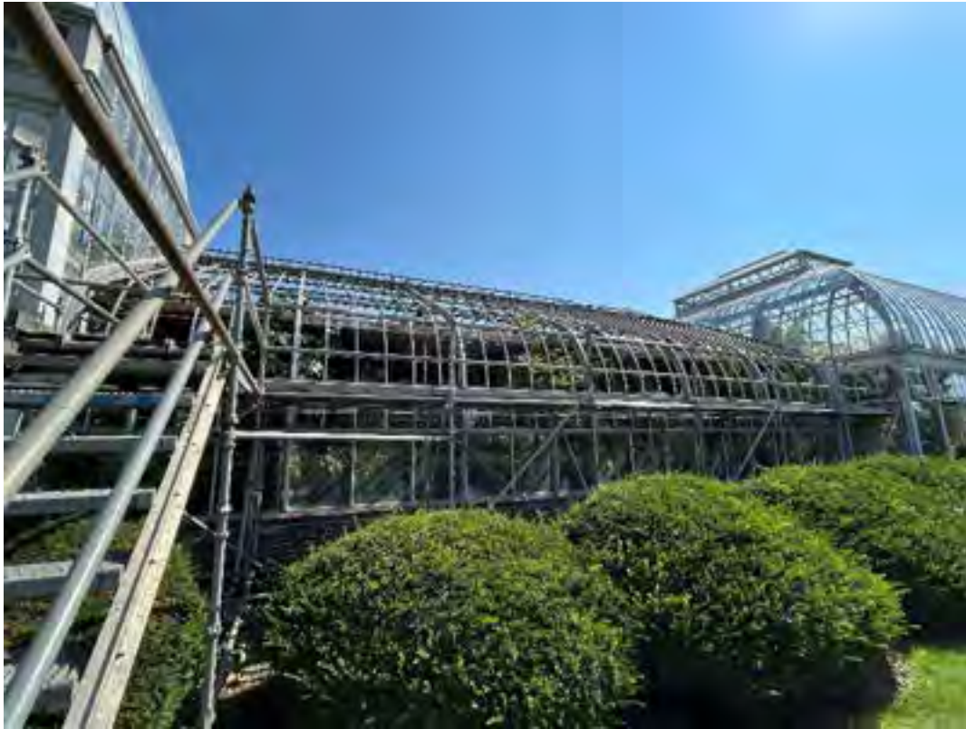
Tropical house with completed glazing and abatement.
