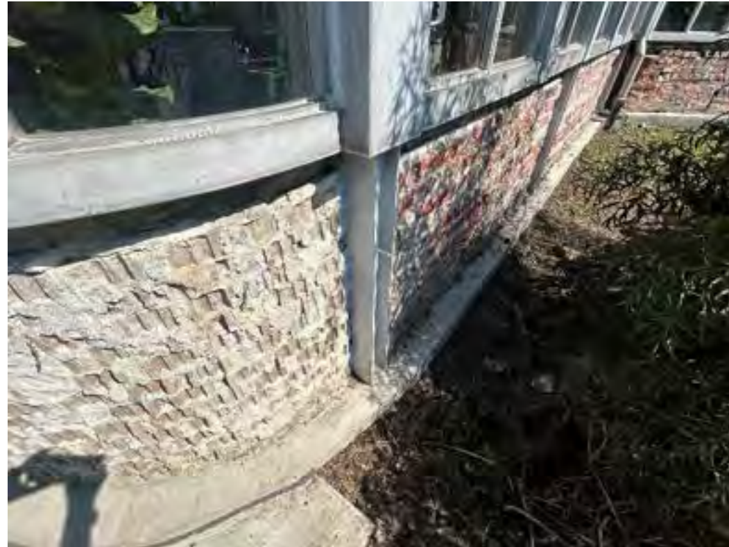
Remaining steel columns all received cleaning and new coating before limestone to be installed.
