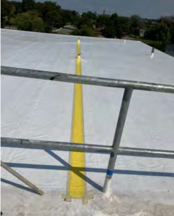
Fall protection installed and safety lines painted.
