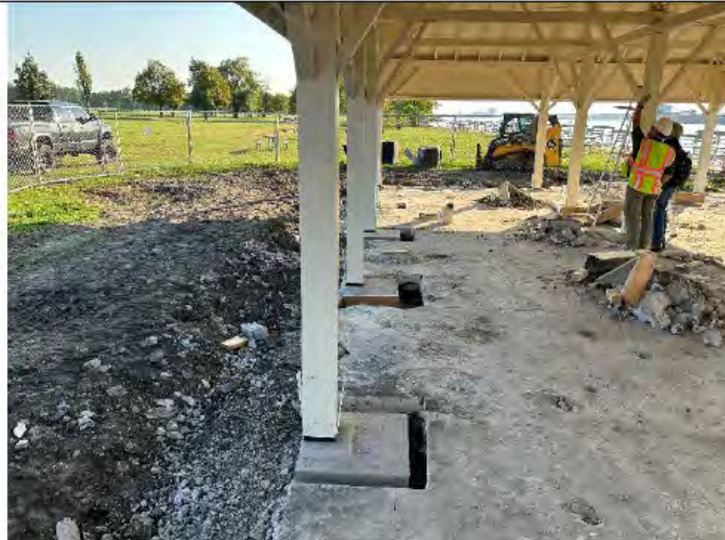
The remaining concrete will all be replaced around the footings..
