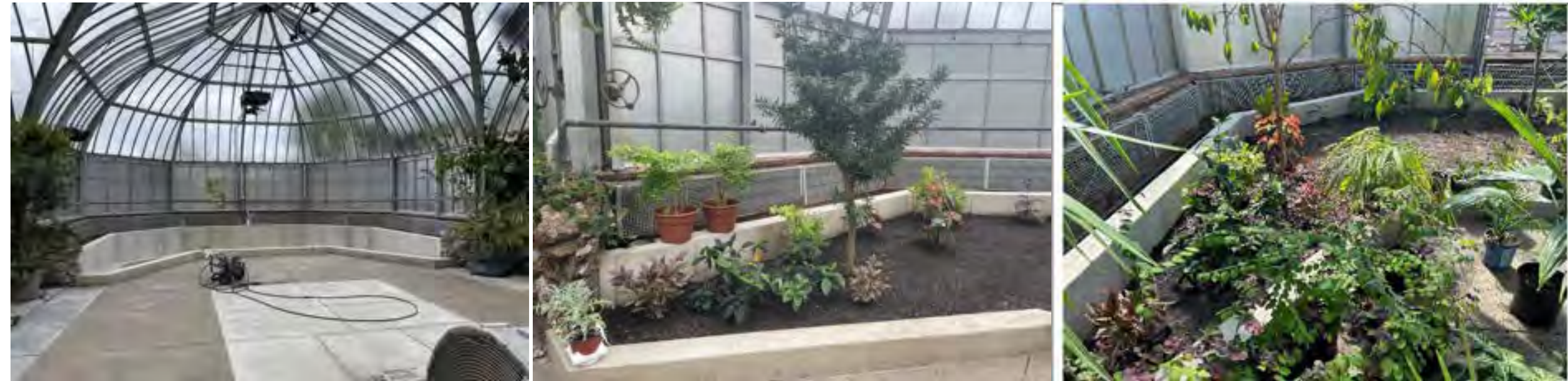
New Planting beds filled with soil and new plantings.
