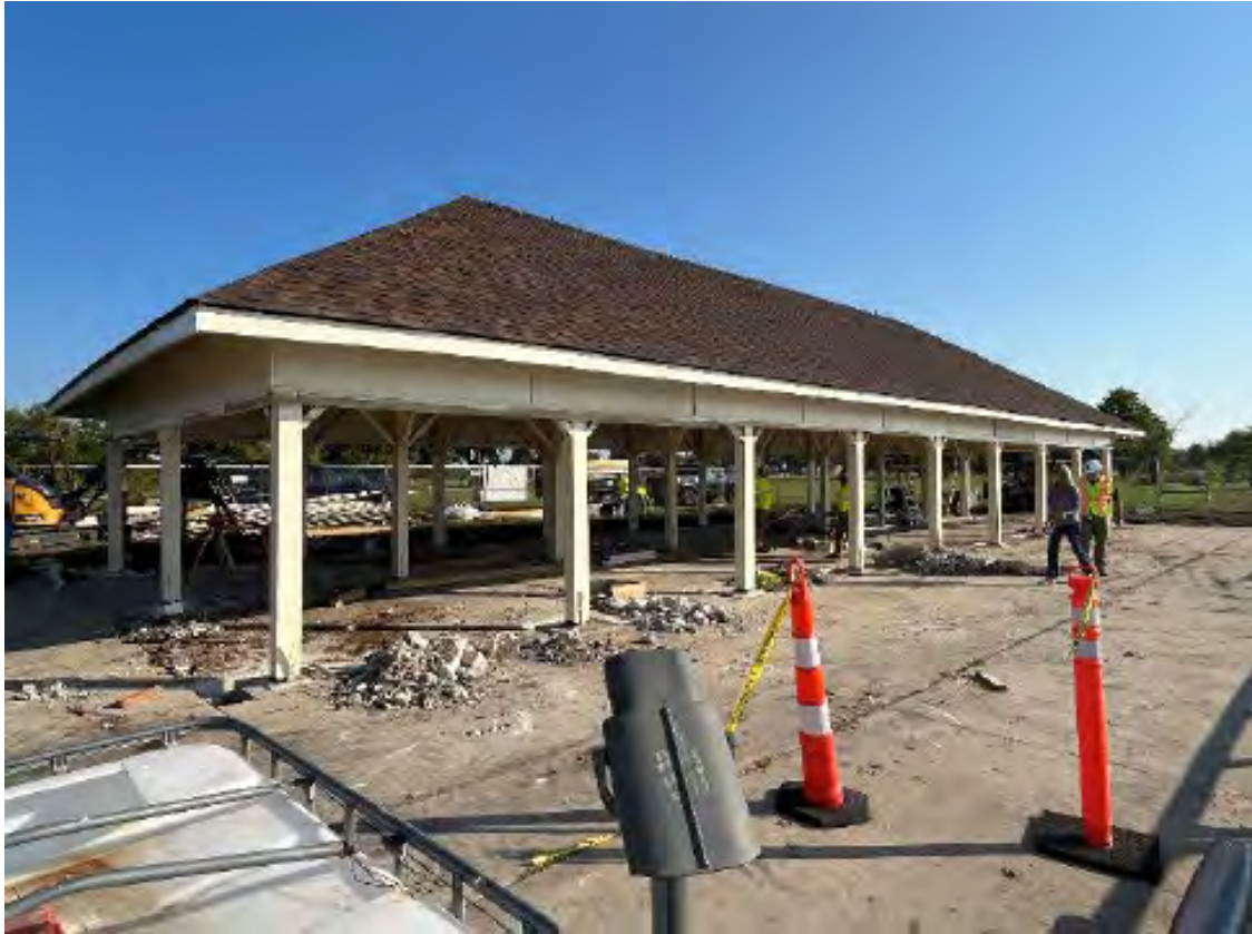
Overview of post replacement.
