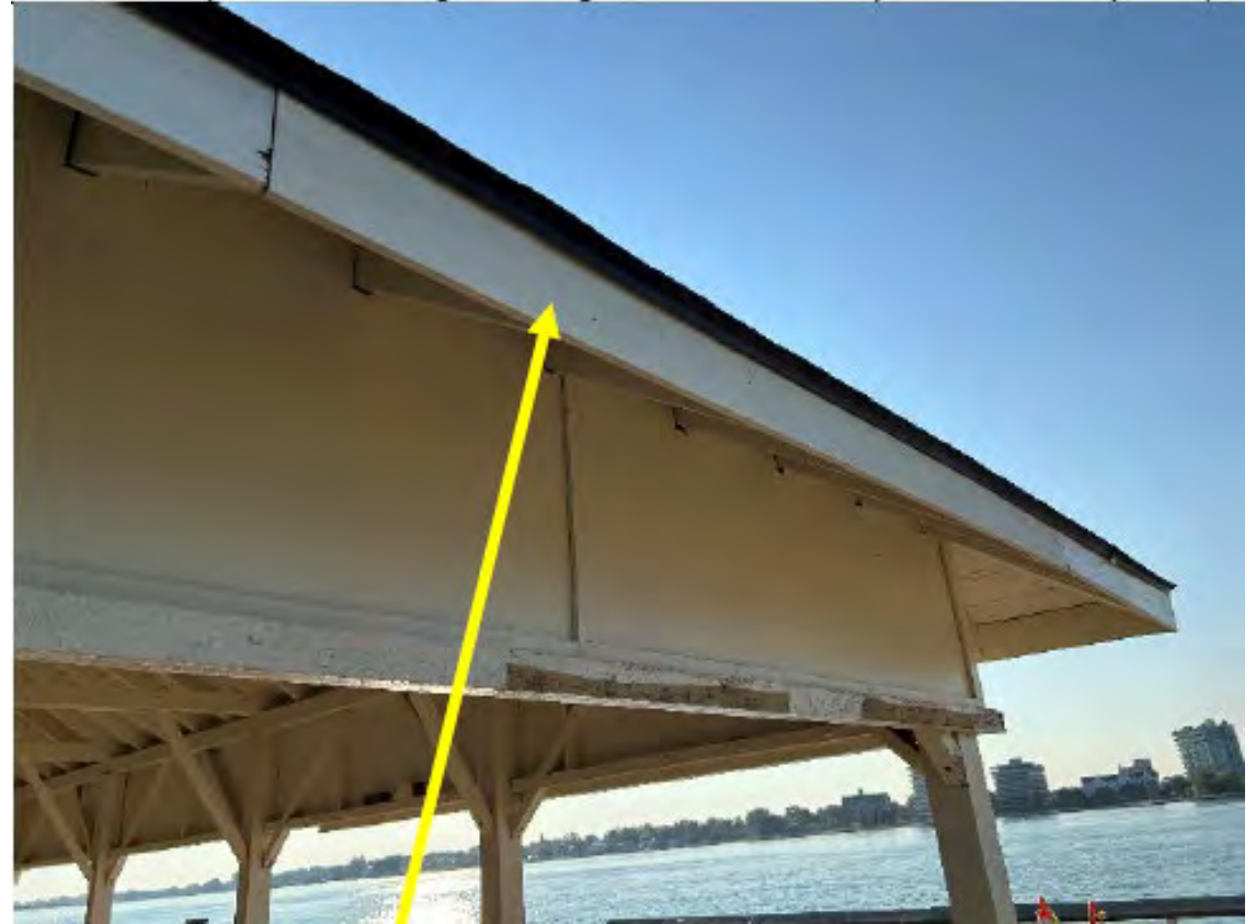
Replaced fascia board.
