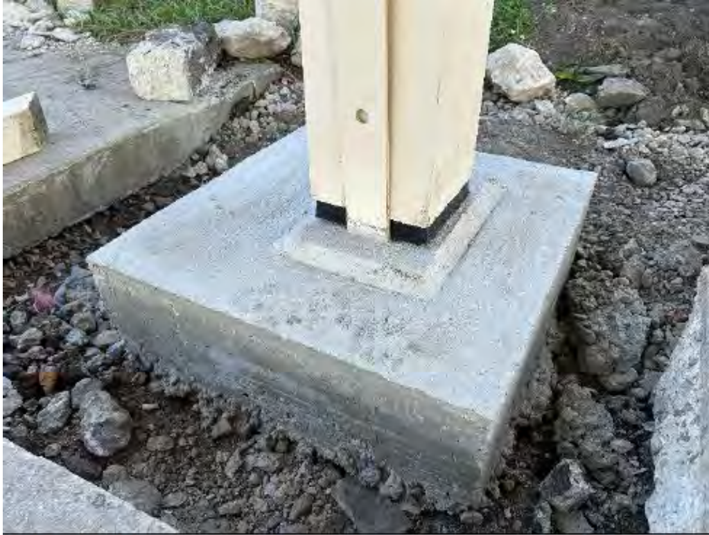
New footings, Post and straps is complete.
