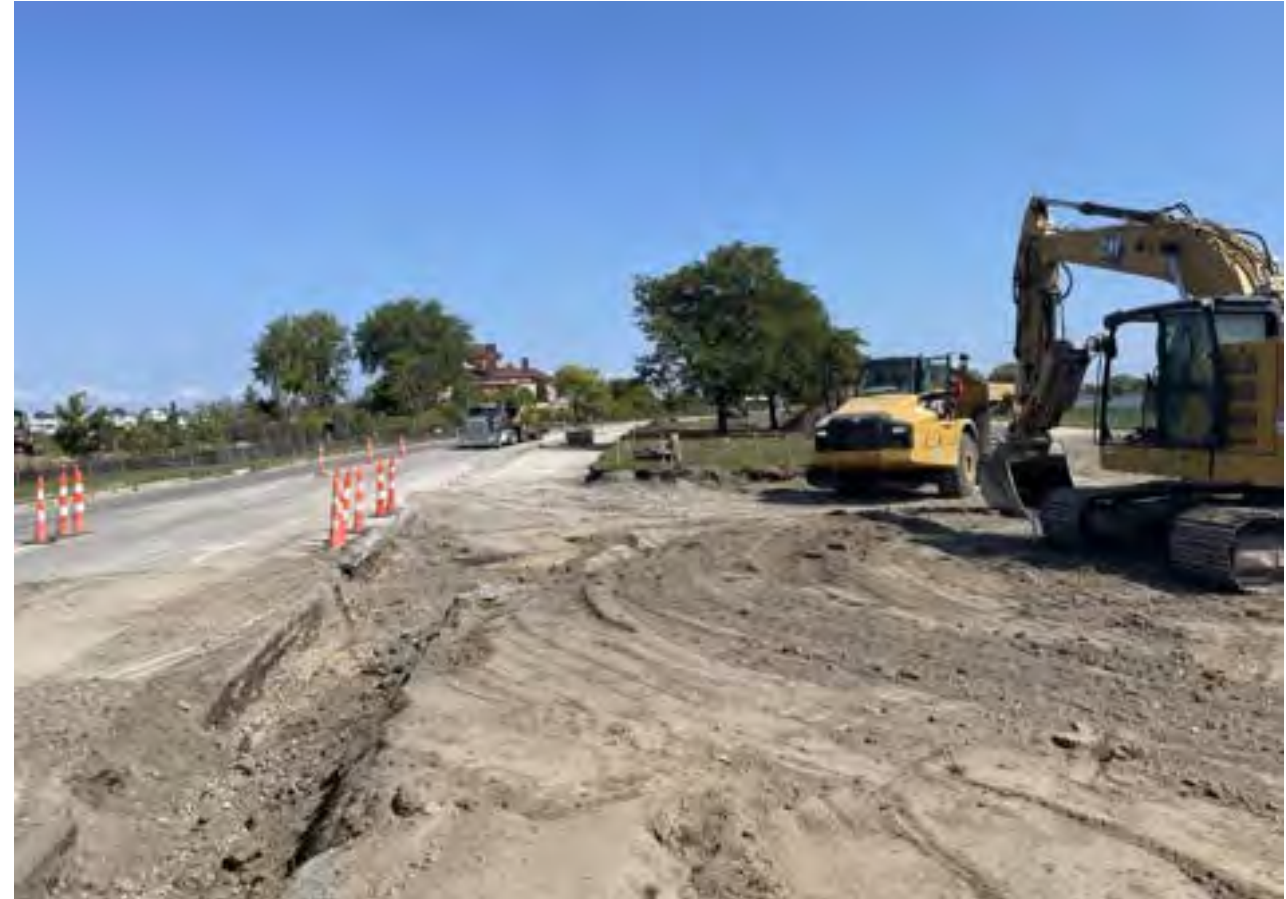
Trail work has begun at the Lake Muskoday Parking lot..
