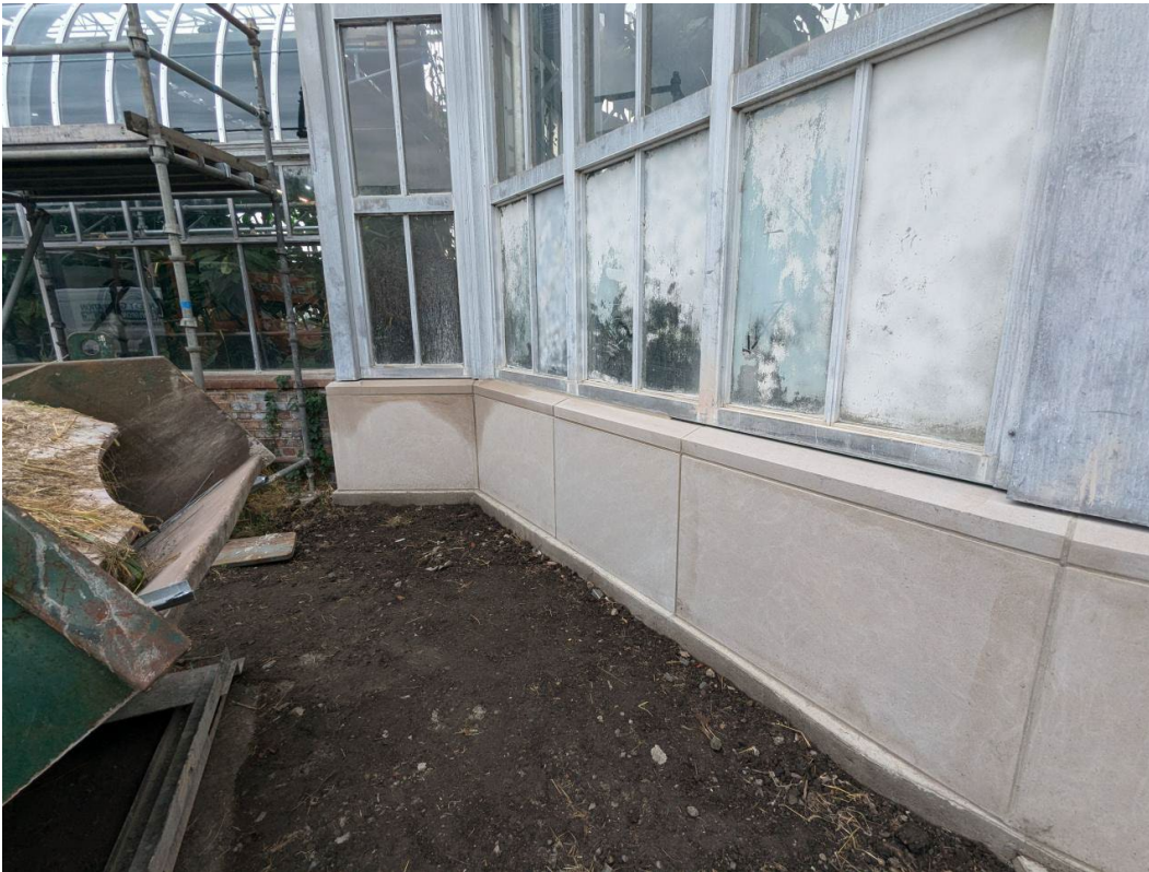
New Limestone Panels and Sill installed; Grading will drain away from wall.
