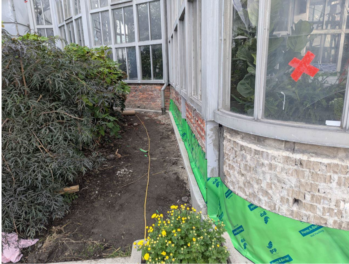
Waterproof membrane in place before new limestone panels to be installed.
