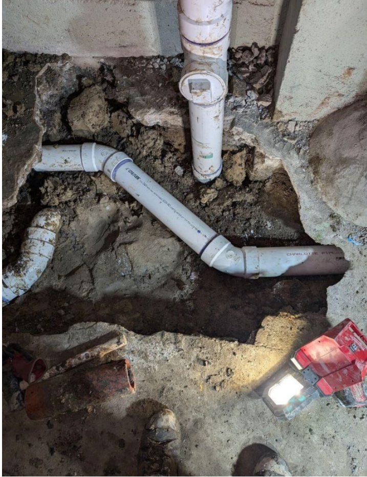
Tying in new storm lines in basement.
